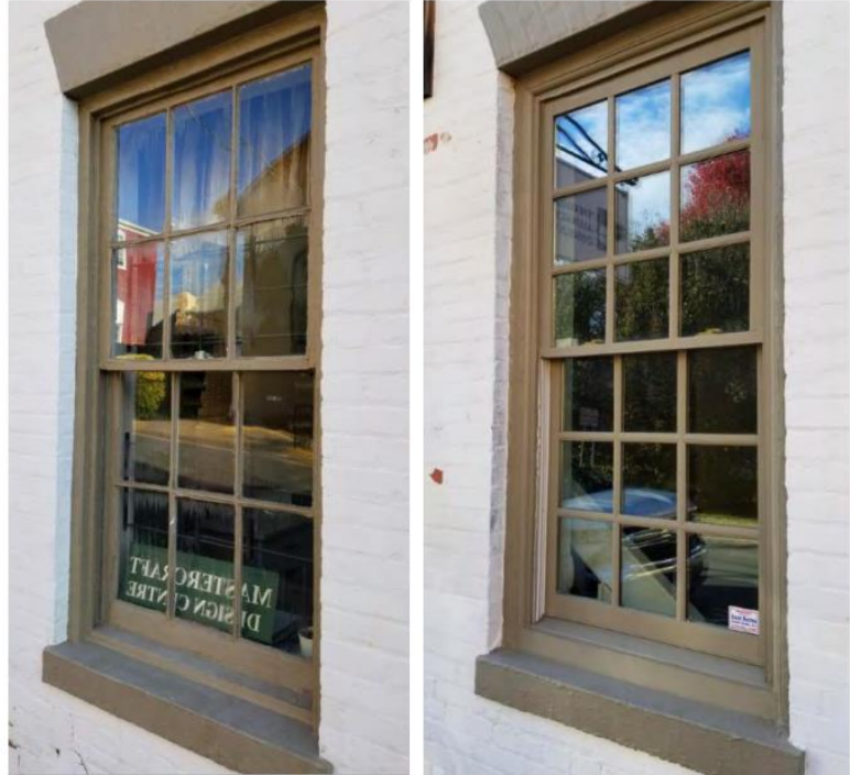
Figure 3-31: The window on right is a wood replacement with moderately accurate detailing. It mimics an original window, as seen on the left. The replacement has slightly thicker muntin profile than the original and also has an incorrect division of lights (nine-over-nine-light as opposed to the original six-over-six-light sashes). Despite these inconsistencies, it is a good fit for the historic district.
