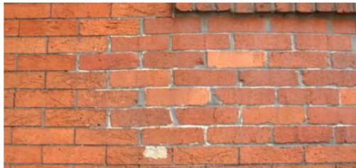
Figure 3-24: This brick wall was improperly repaired; the replaced mortar does not match the existing mortar profile, color, composition, or texture. Further, an improper re-pointing technique damaged the brick.
