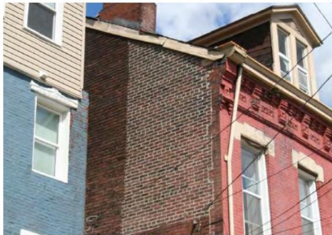
Figure 3-25: Do not re-point masonry joints with a mortar that does not duplicate the old in strength, composition, color, and texture, as pictured above. Whether original to the house or added at a later date—the appropriate design minimally affects the integrity of the house.
