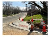
• Removed and replaced a section of sidewalk where the roof drain pipes go through. The section was crumbling and had become a trip hazard to pedestrians.
