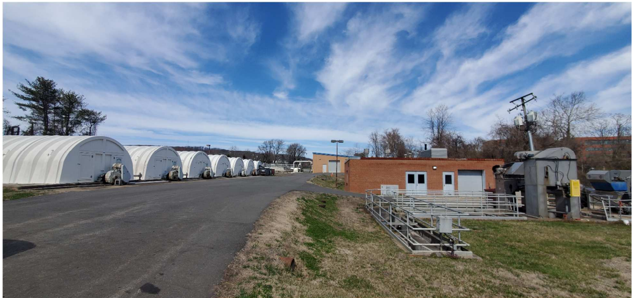
NORTHERLY VIEW ACROSS SUBJECT FROM NEAR SUBJECT’S SOUTHERN PROPERTY LINE ENTRANCE.
