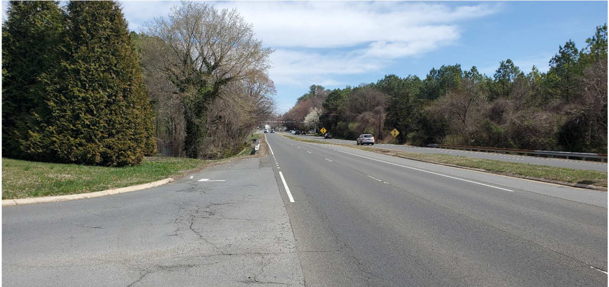
EASTERLY VIEW ALONG FROST AVENUE (RT. 211) FROM THE ENTRANCE FOR THE “WHARF” PROPERTY INGRESS/EGRESS EASEMENT. SUBJECT NOT VISIBLE.
