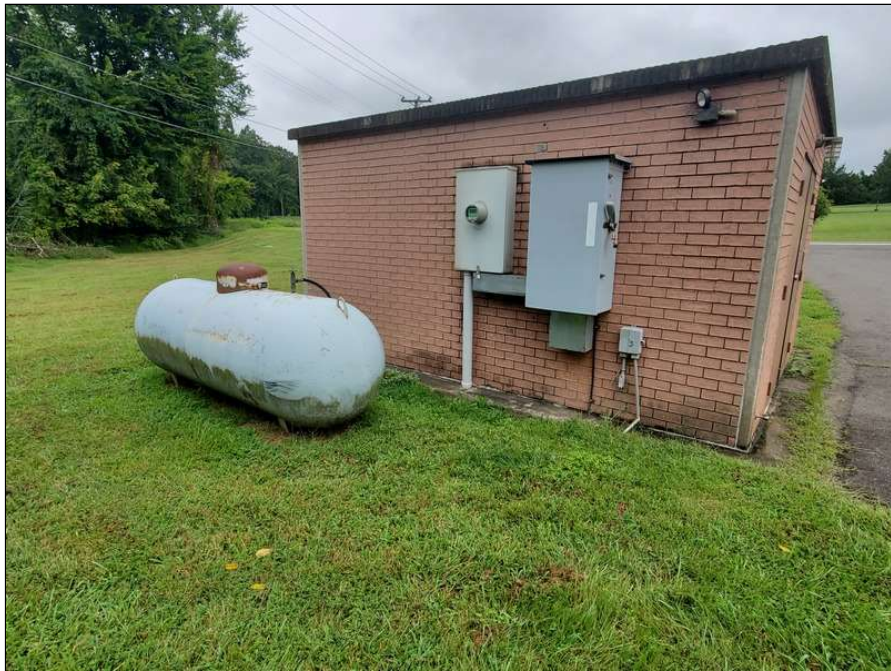
8 - Rear of utility shed
