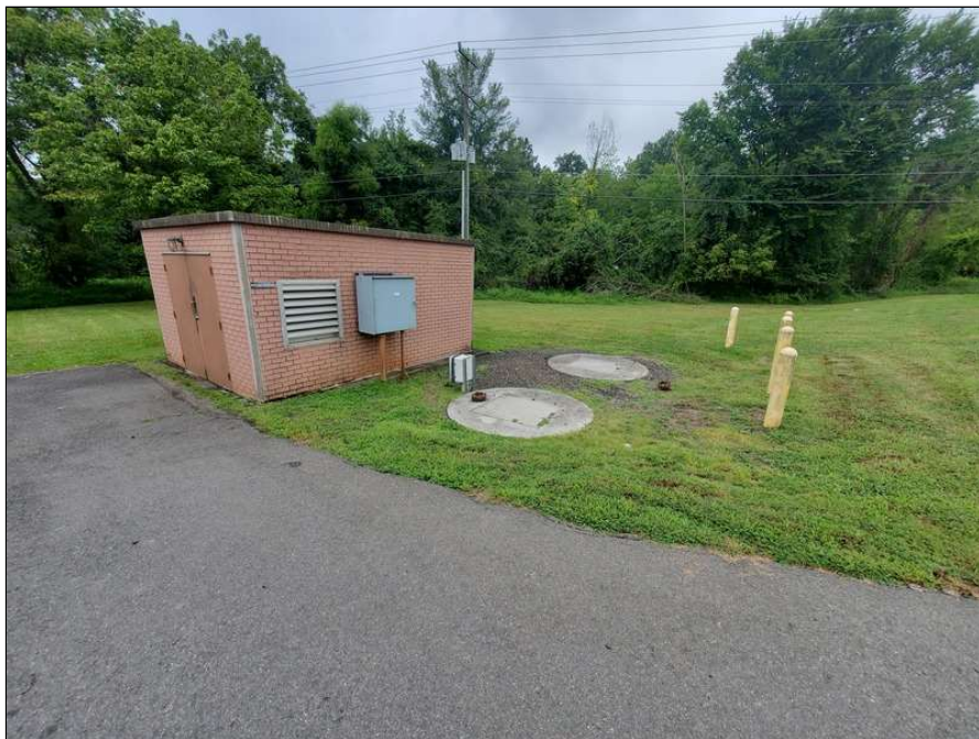
10 - Small utility shed/pumping station on northwest portion of site
