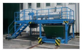
Outdoor installation of a HUBER Sludgecleaner STRAINPRESS®
