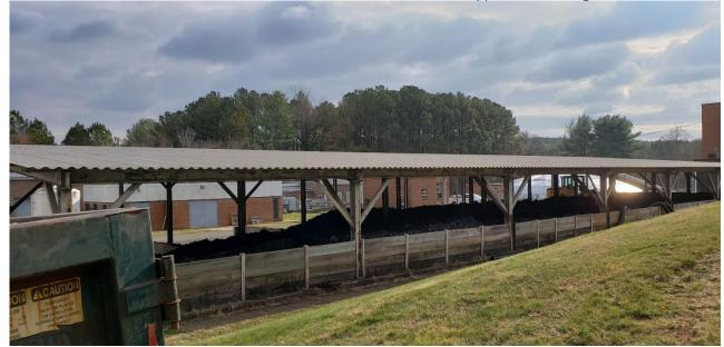
4. Along the front of the sludge storage area, the openings for each bay of the short concrete wall were cut after the fact, based on observations of exposed rebar ends and aggregate at the edges of the walls. We recommend parging the cut ends of each wall with a patching mortar to smooth the wall edges and to protect the steel reinforcement.
