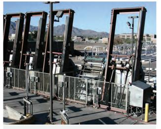
The tougher functionality of the Duperon<sup>®</sup> FlexRake<sup>®</sup>, proven through repeated grease attacks and high I & I, was just one benefit of the equipment's installation in Phoenix, Arizona. During plant upgrades, the low profile of the Duperon<sup>®</sup> FlexRake<sup>®</sup> saved over \$1M in construction costs when compared to previous equipment.
