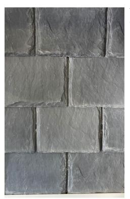
To the left is a close-up of the shingles as they would appear installed on the roof of my smokehouse.
