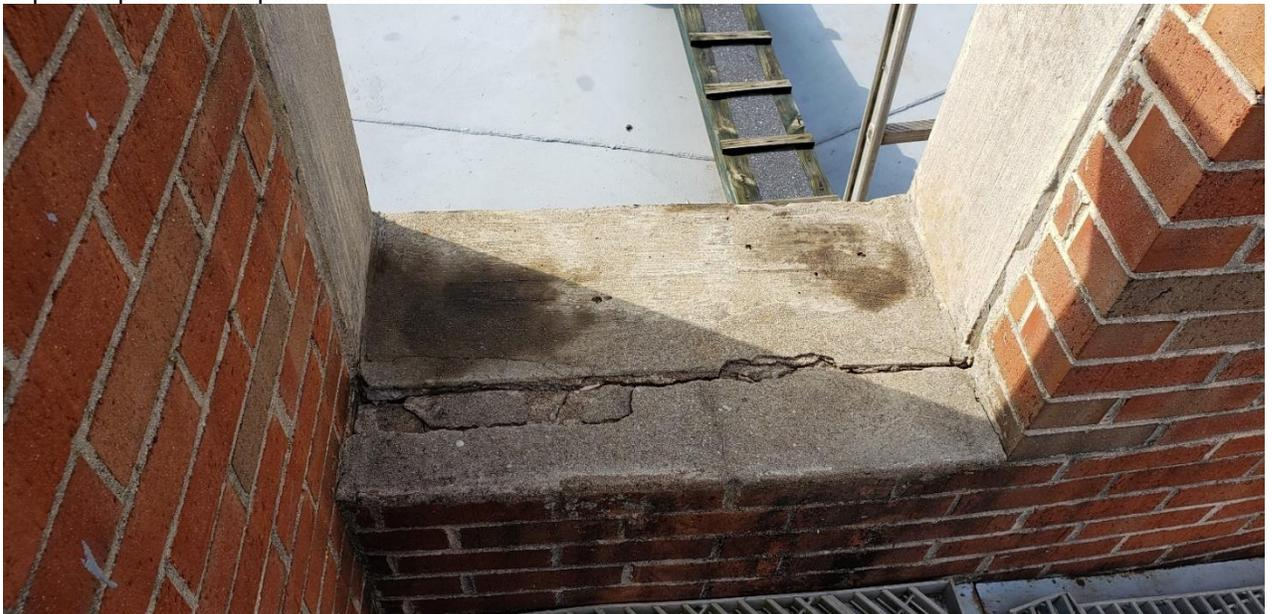
11. The concrete brick shelf corbel extending from digester walls was exposed in several locations around the perimeter of the building. Typically this brick shelf would be below grade so the bottom of the brick façade would terminate below grade where it would not be seen. The visible brick shelf is primarily a cosmetic deficiency; however, the fact that so much of the brick shelf is exposed could be evidence of grading erosion caused by slope stability issues of the steeply-sloped grade.
