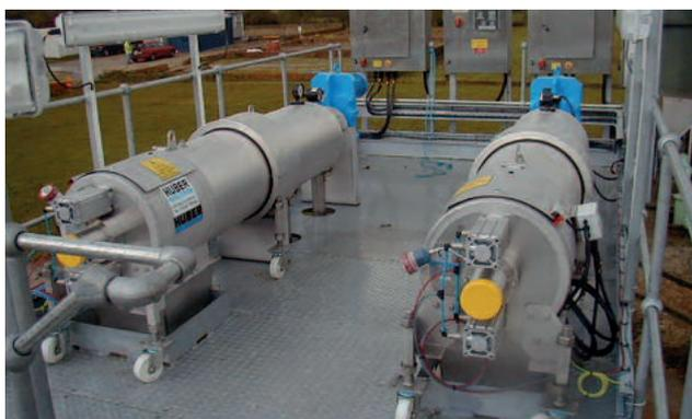
*STRAINPRESS® with heatable casing pipe*
