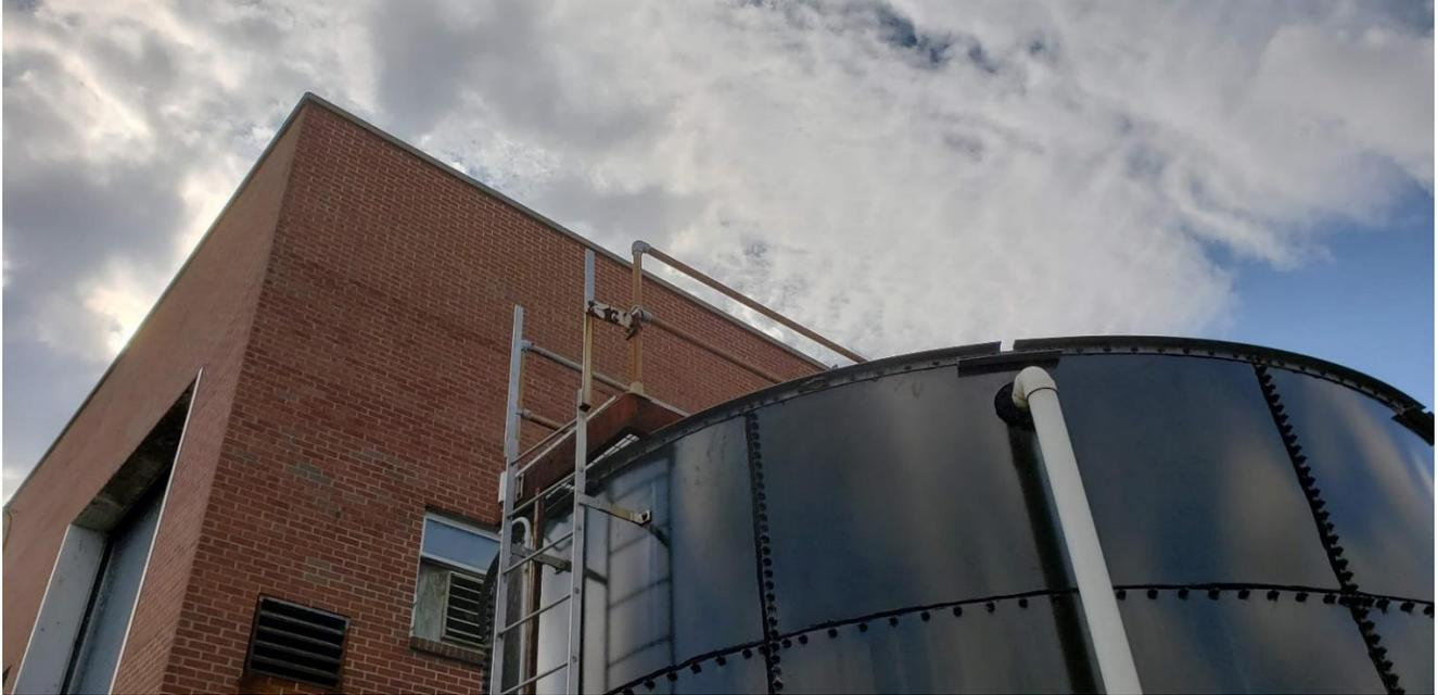
5. North Elevation: The louver on the north elevation is rusted. Recommended to remove louver and replace in kind. Clean rust stains from brick façade.
