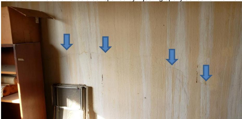
2. A long vertical hairline crack observed on circular wall of digester tank, extending from Upper Level slab to roof slab. This crack should be repaired by injecting epoxy adhesive into the crack.
