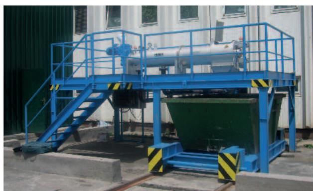
*Outdoor installation of a HUBER Sludgecleaner STRAINPRESS®*
