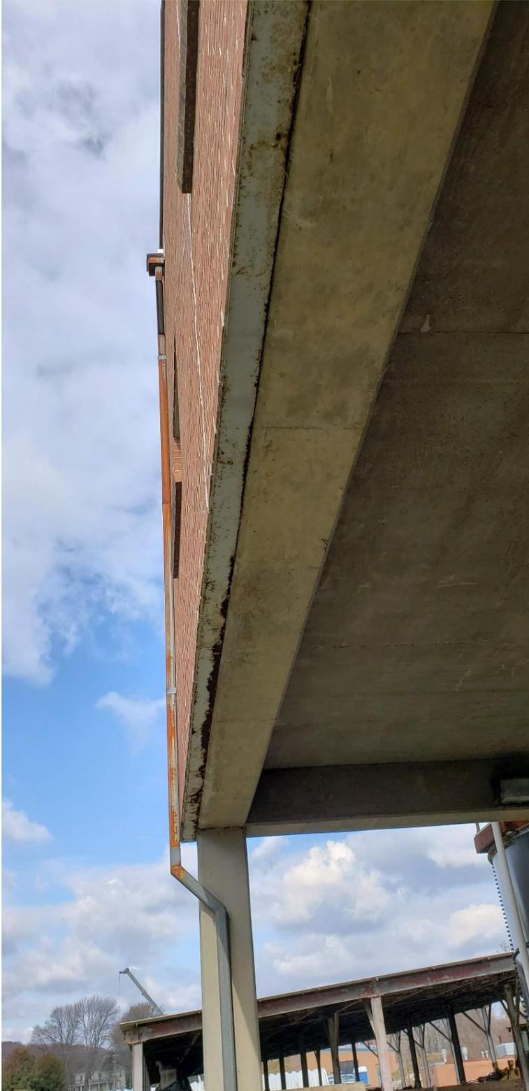
3. The two downspouts from high roof scuppers are rusted. Recommended repair is to remove existing downspouts and replace in kind.
