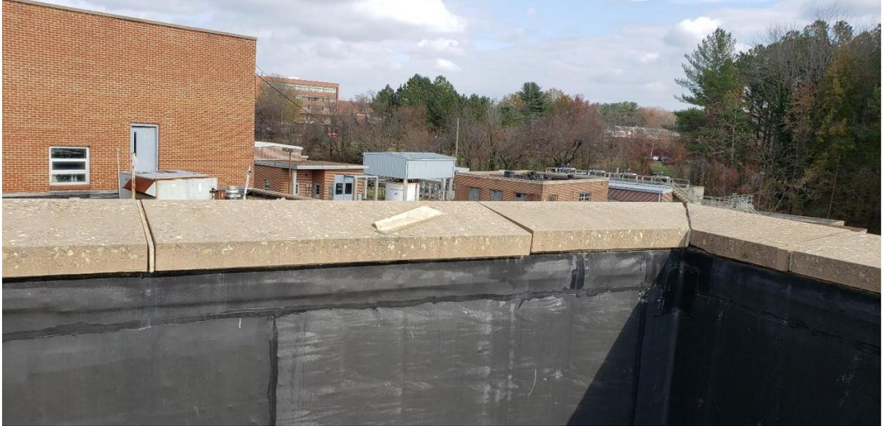
10. Cracking and spalling was observed at the wall opening to access the top of the digester from the exterior. Crack aligns with the joint between the digester concrete wall and the brick façade. Recommended repair is to patch spalls with repair mortar and to route and seal the crack.
