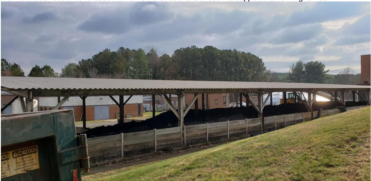
4. Along the front of the sludge storage area, the openings for each bay of the short concrete wall were cut after the fact, based on observations of exposed rebar ends and aggregate at the edges of the walls. We recommend patching the cut ends of each wall with a patching mortar to smooth the wall edges and to protect the steel reinforcement.
