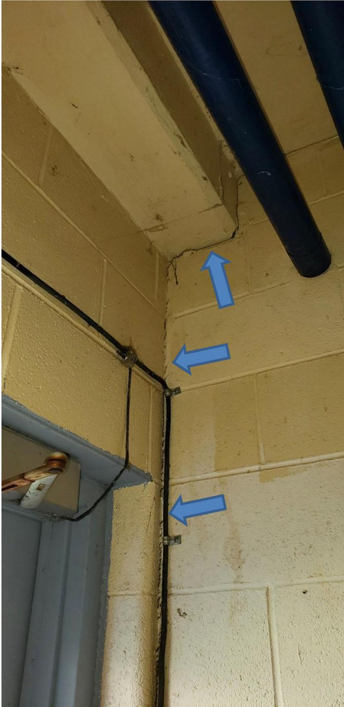
5. Hairline cracks were observed in Upper Level slab between valve operator floor stands. These cracks should be repaired by injecting epoxy adhesive into the cracks.
