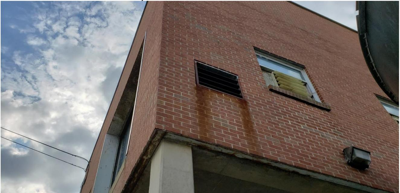
6. East Elevation: Top of brick veneer has spalled under concrete sill at Second Floor overhead door. Recommended to remove damaged bricks and replace in kind, then seal joint between concrete sill and brick below with a flexible joint sealant and backer rod.
