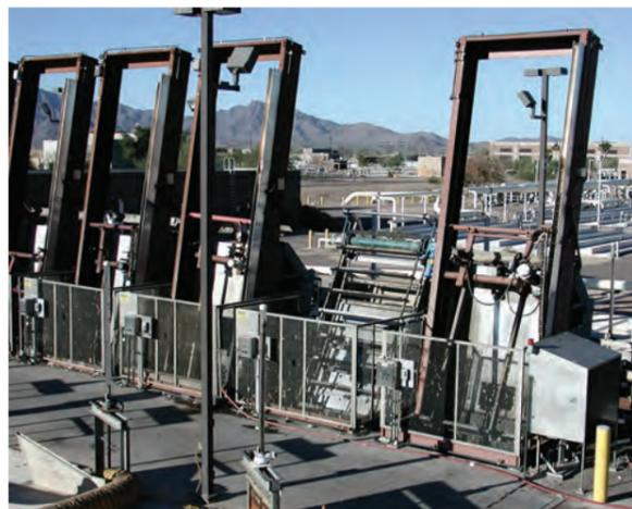
The tougher functionality of the Duperon® FlexRake®, proven through repeated grease attacks and high I & I, was just one benefit of the equipment's installation in Phoenix, Arizona. During plant upgrades, the low profile of the Duperon® FlexRake® saved over \$1M in construction costs when compared to previous equipment.
