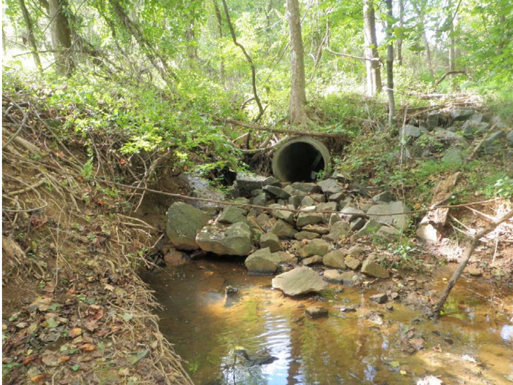
Photo 5 – Looking upstream at discharge pipe from SWM device.
