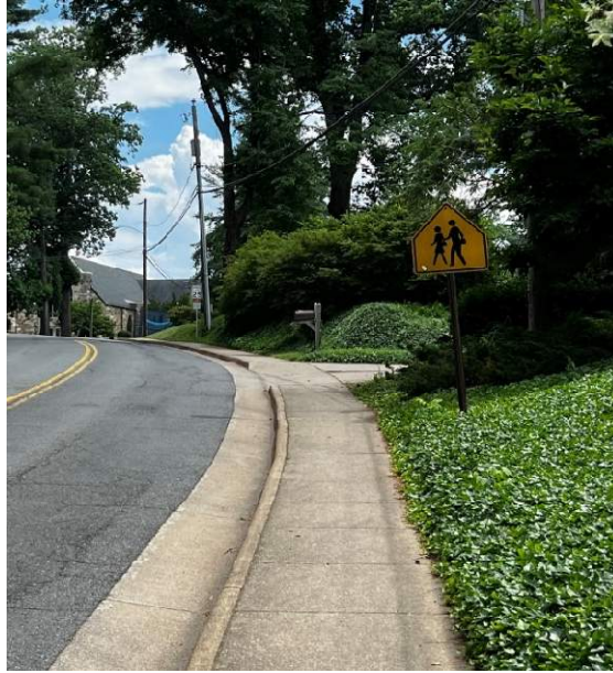
Figure 10. Existing Signage in Study Area - Signage without retroreflectivity on northbound Winchester Street, north of St. John School Driveway
