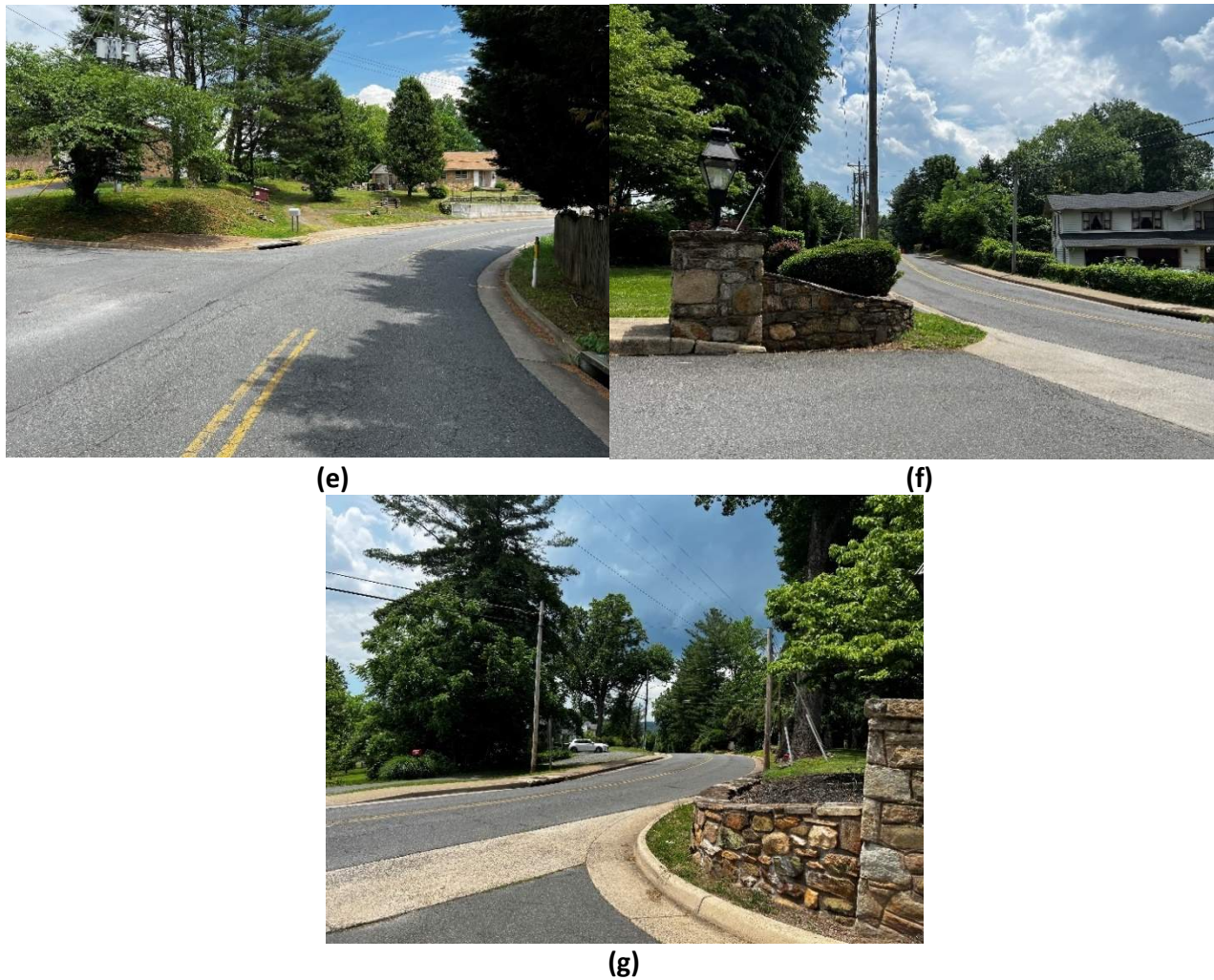
Figure 9. Limited Sight Distance in Study Area
