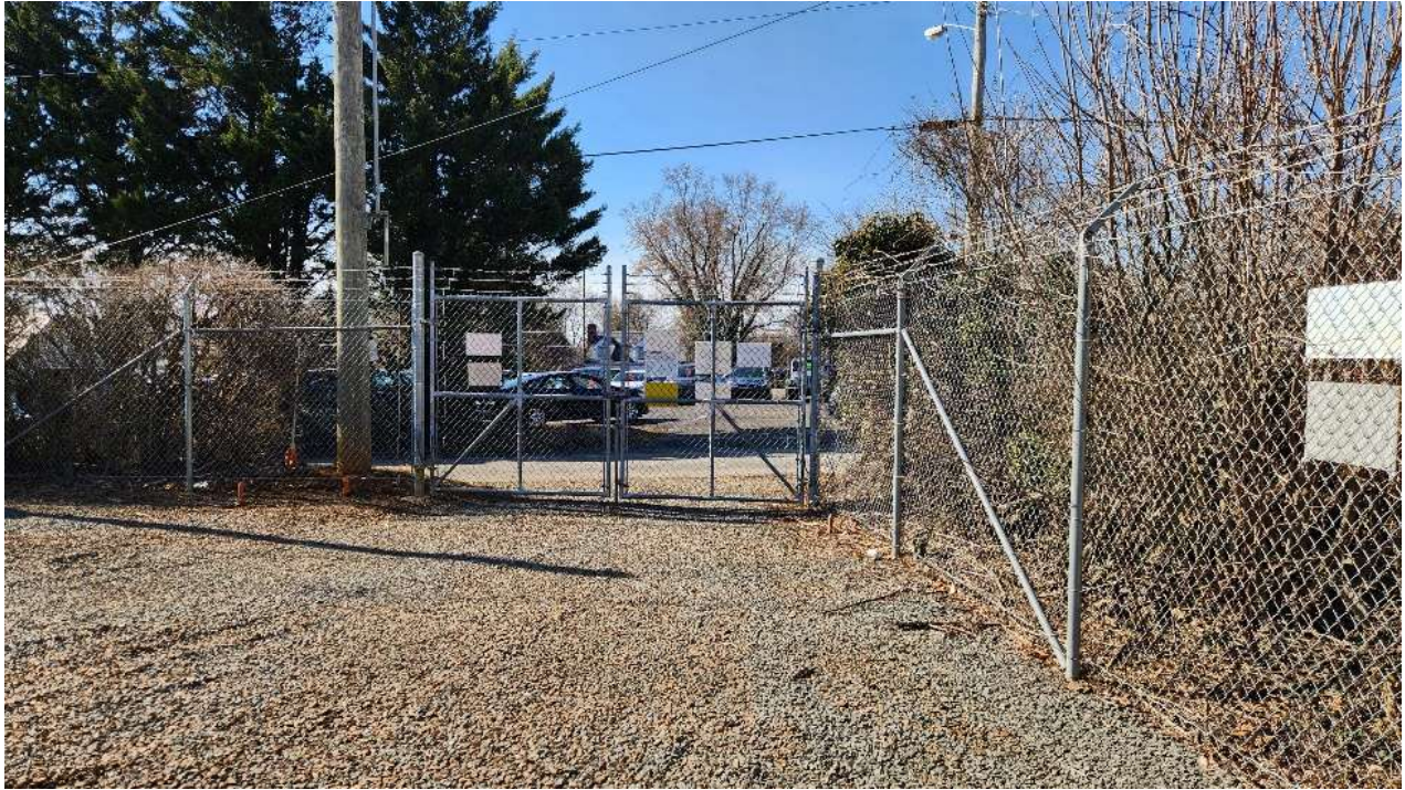
Example photo of existing security fence
