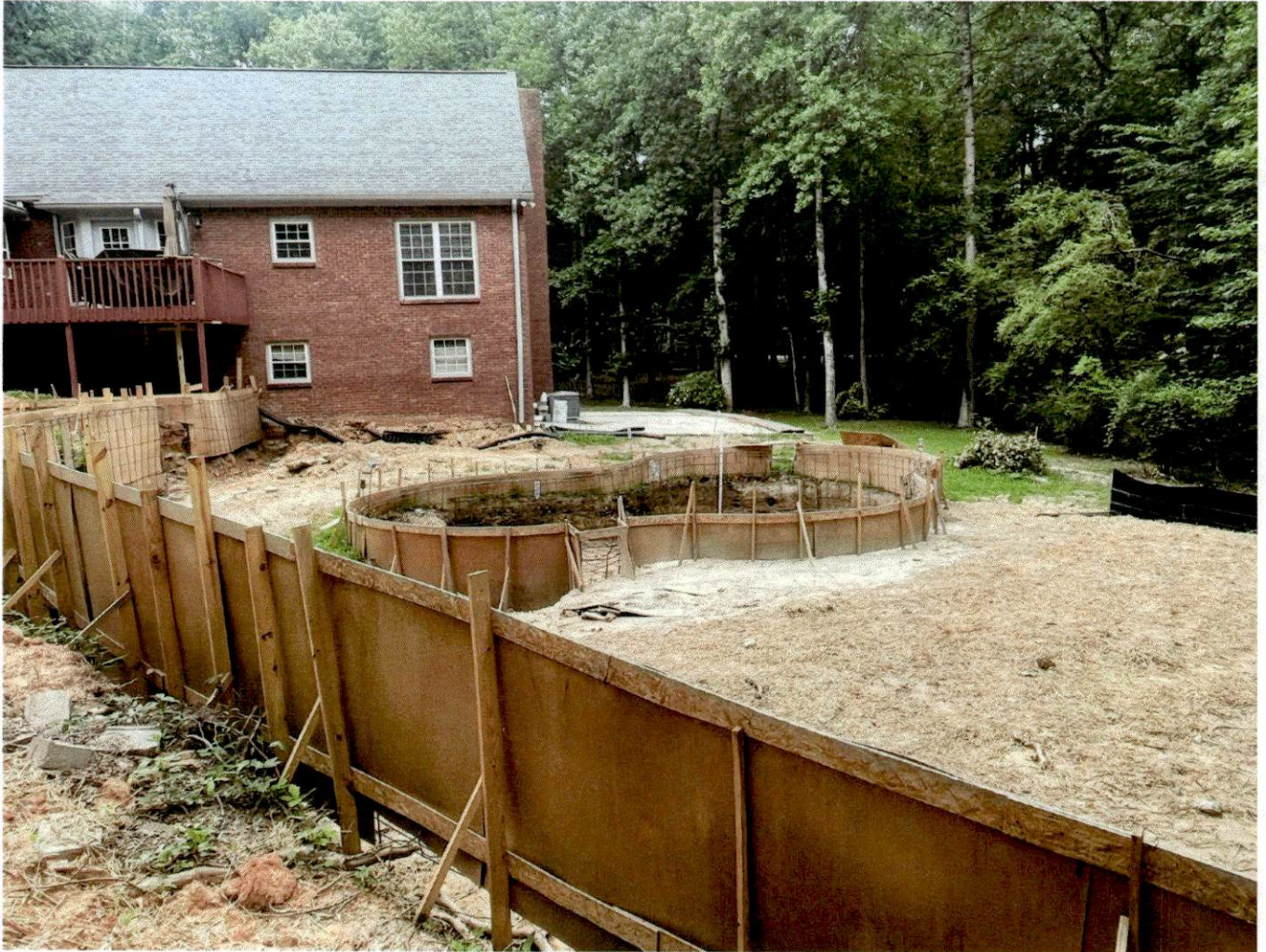
View of retaining wall and back side of the pool.
