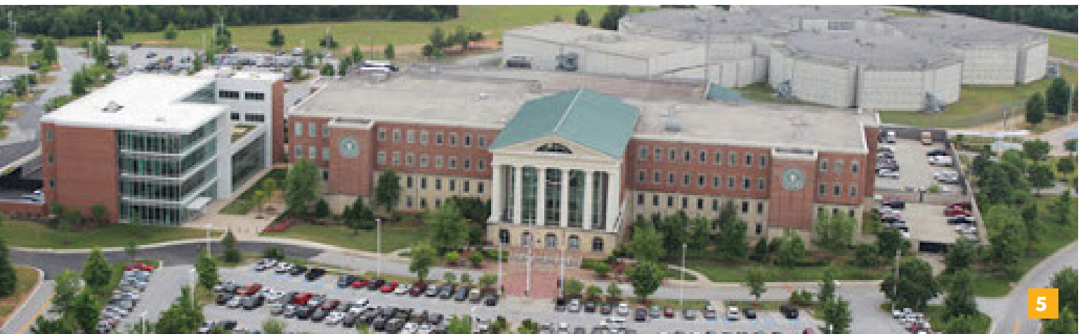
1. Adult Detention Center Campus - Cobb County; 2. Adult Detention and Law Enforcement Center - Douglas County; 3. Adult Detention and Law Enforcement Center - Paulding County; 4. Adult Detention and Law Enforcement Center - Carroll County; 5. Adult Detention and Law Enforcement Center - Clayton County; Project Profiles for highlighted projects above are provided on the following pages.
