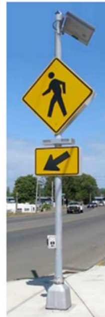
Wrap-around RRFB Light Bar with Required Signage
