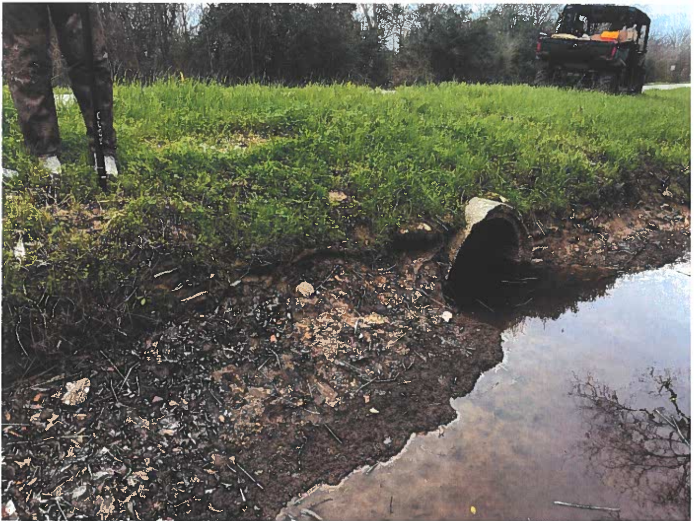
Figure 3. View of culverts on west side of Penick Road. Note the top edge of the blocked culvert is visible in the center of the photo, with the active culvert to the right.
