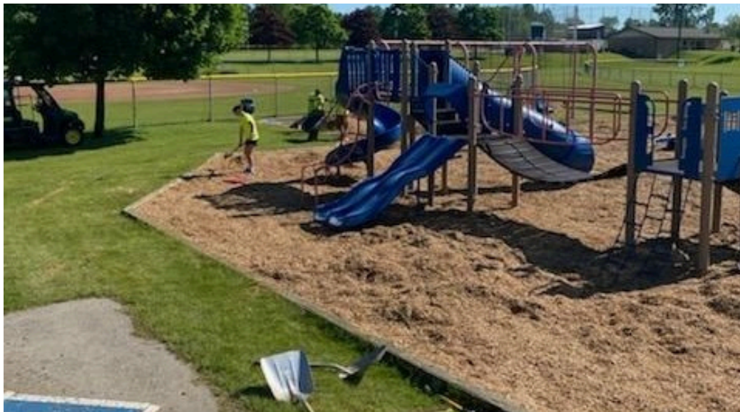
New mulch being installed at the playground.
