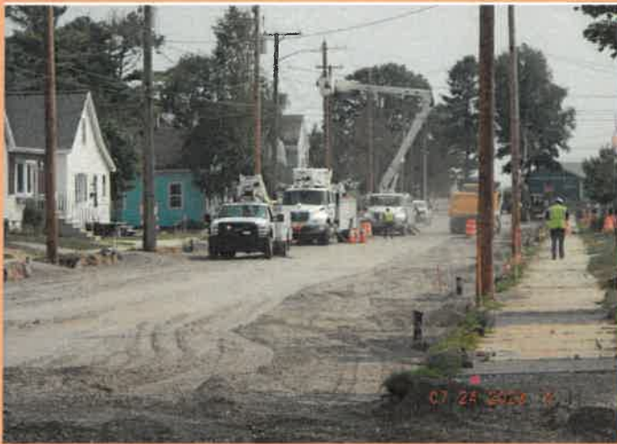
Lincoln Street utility work, storm sewer installation and grading and gravelling
