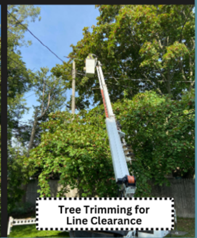
Tree Trimming for Line Clearance
