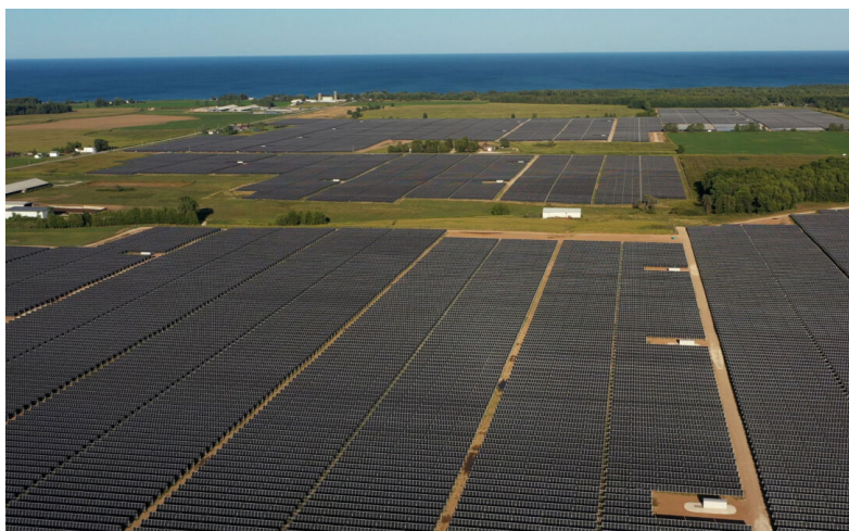
Point Beach Solar Energy Center
