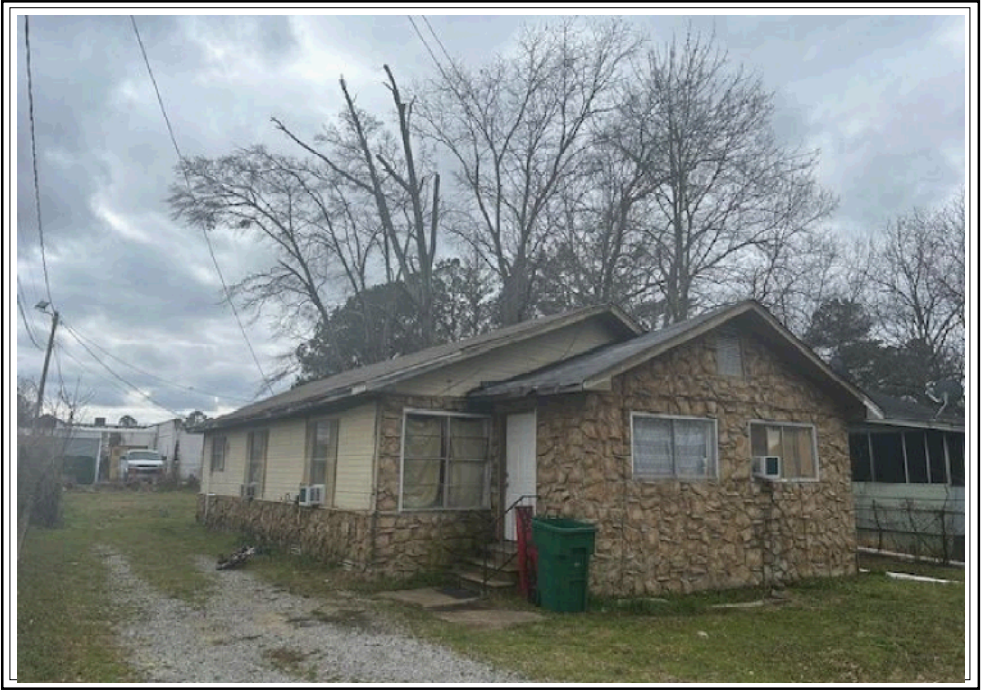
FRONT VIEW OF SUBJECT PROPERTY
