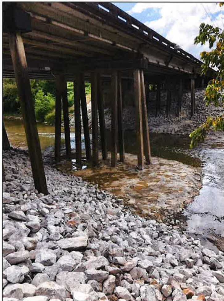
Bridge Piers after Rip Rap and Grouting to prevent erosion in the future
