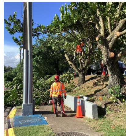
Ceres Performing Work for the LUMA Vegetation Clearing Services Contract
