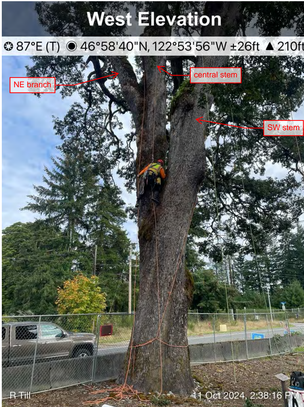
Figure 1 Inspection of first codominant union. A ¼ inch steel probe was inserted between stems and encountered solid resistance below historic debris collecting between the stems.
