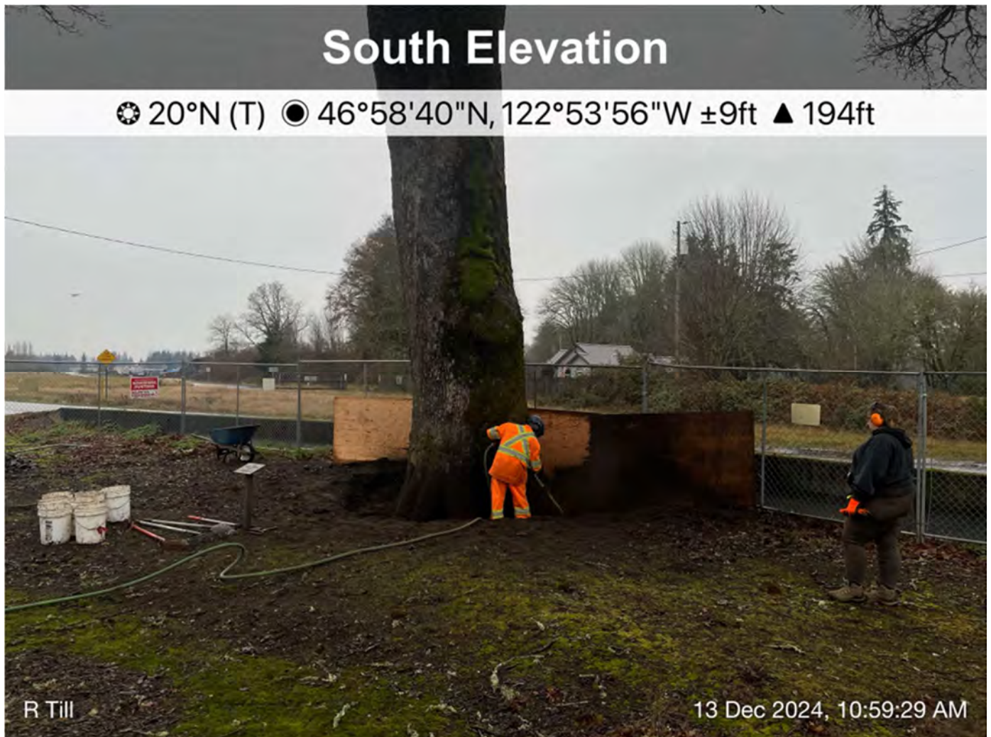
Figure 1 Root crown excavation employed an “air spade” that uses compressed air to remove fine soil. The excavation involved alternating between air spade removal of soil with hand removal of river cobble that was backfilled over the root flare after a prior root crown excavation. The project archaeologist oversaw all work.
