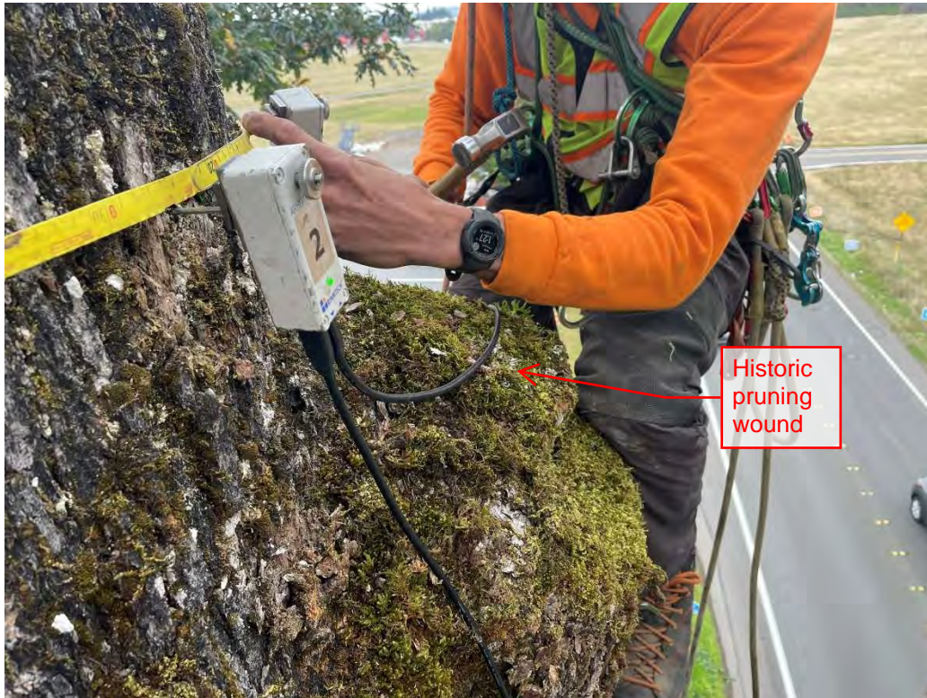
Figure 14 Historic pruning wound (covered in moss directly below watch) approximately 1 foot above the 2023 failure and below the Kestrel cavity.
