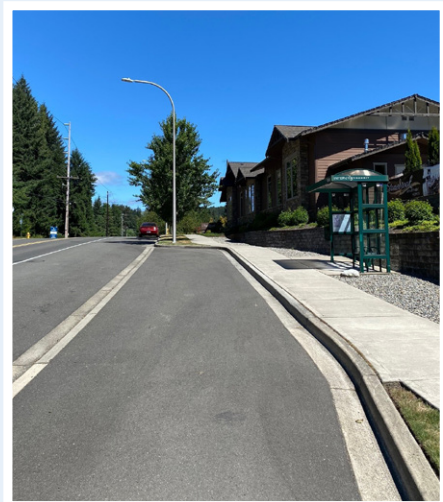
Pull-out bus stop on Rural Rd. at 48th Ave., northbound
