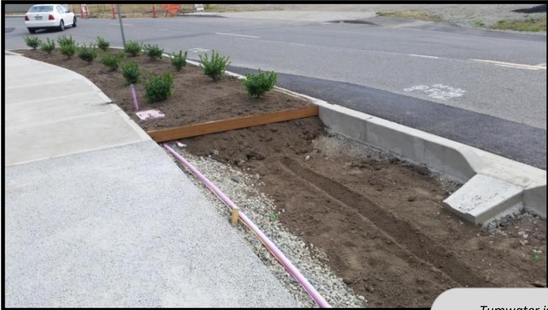
*Tumwater is employing new Low Impact Development techniques – such as this infiltration baffle shown under construction on Linderson Way – to reduce the effects on the environment of stormwater runoff.*
