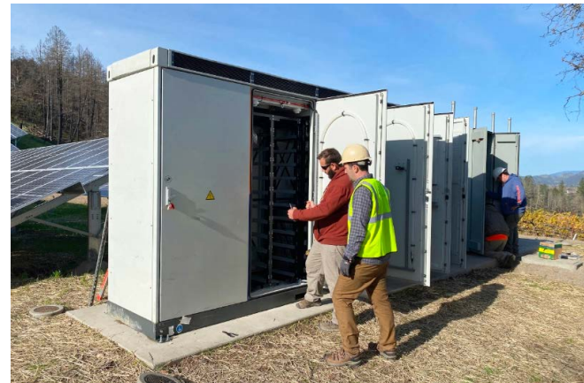
Example of a Containerized BESS Unit
