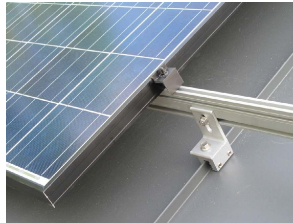
Examples of Mounting Systems for Standing Seam Metal Roofs.
