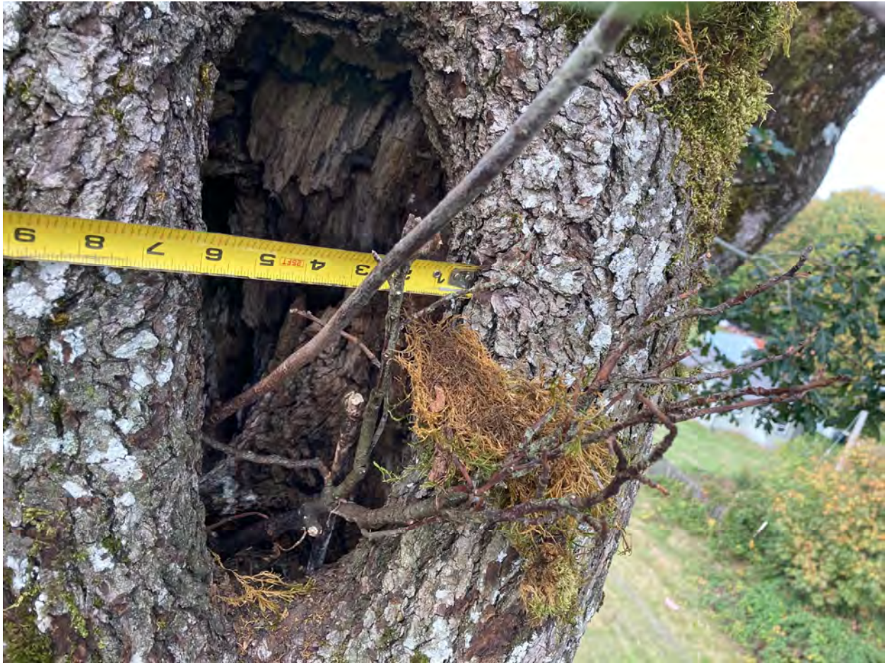
Figure 20 Measurement of diameter of cavity at 6 inches.
