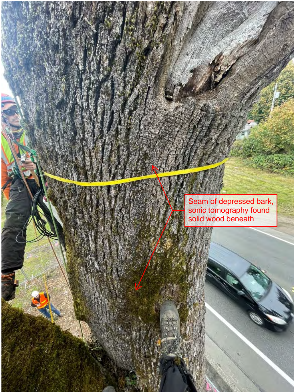
Figure 5 Seam below 2012 failure. Sonic tomography found solid wood down into codominant union.
