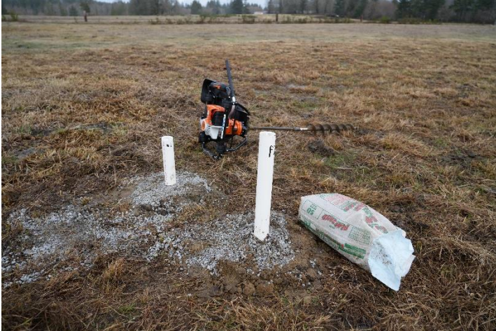
Photo 43. Installing Well W1 and Piezometer P1
