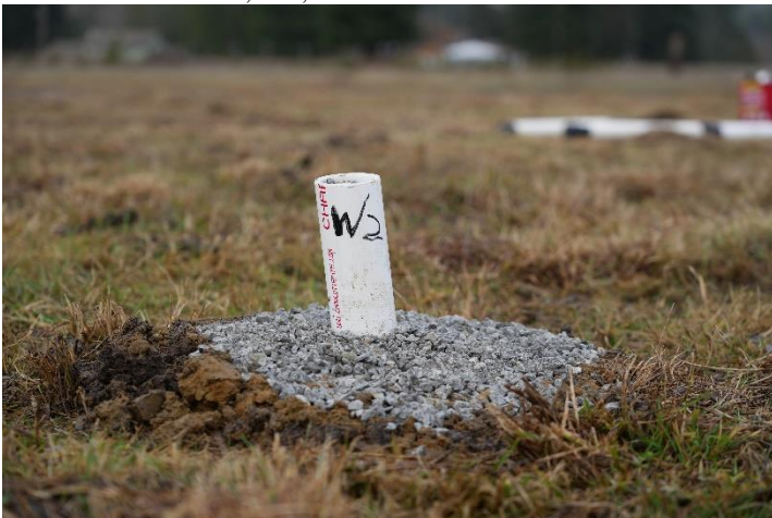
Photo 47. Well W2 in Area A
