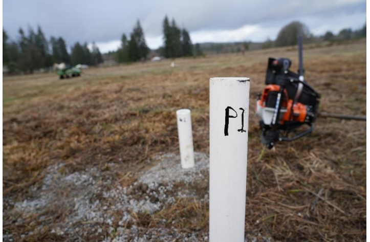
Photo 44. Installing Well W1 and Piezometer P1
