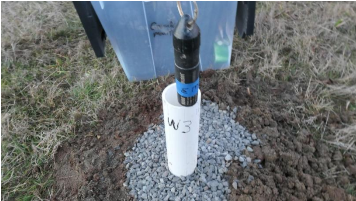
Photo 51. Datalogger in Well W3
