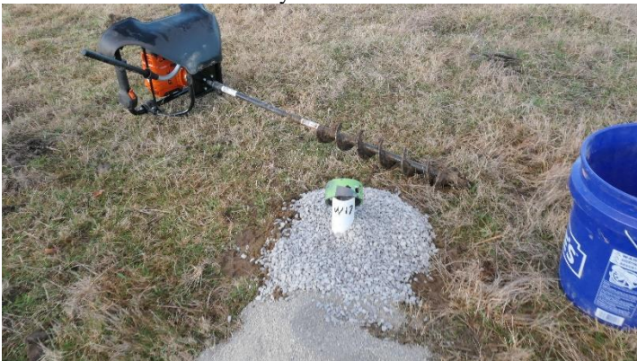
Photo 75. Installation of Well W17 in Study Area F
