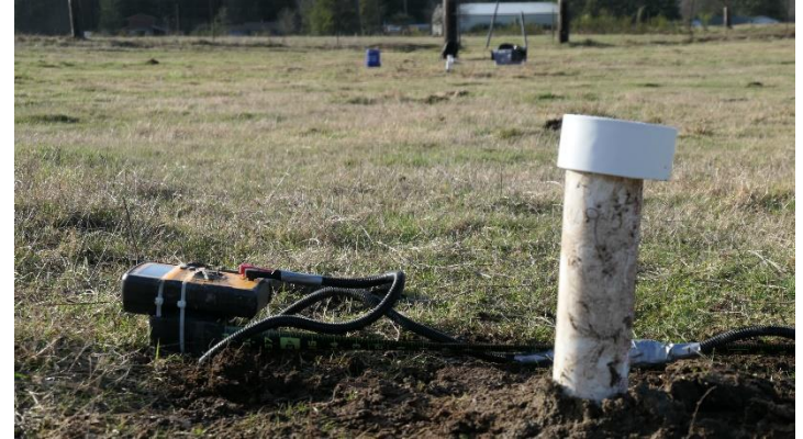
Photo 60. Device to measure water depth in well
