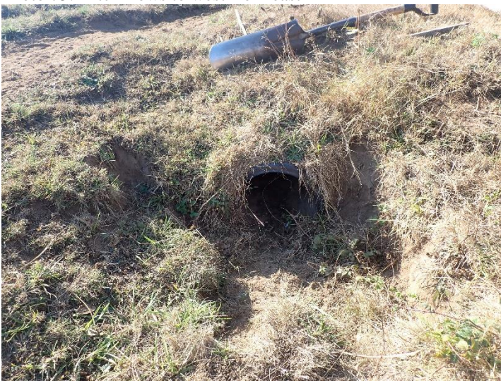
Photo 77. Culvert under crossing of east-west ditch
