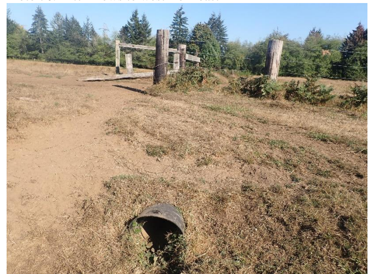
Photo 78. Culvert under crossing of east-west ditch
