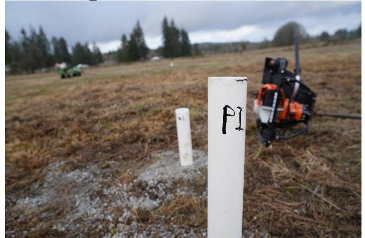
Photo 44. Installing Well W1 and Piezometer P1
