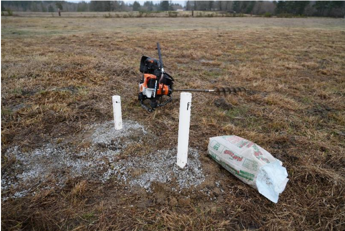
Photo 43. Installing Well W1 and Piezometer P1
