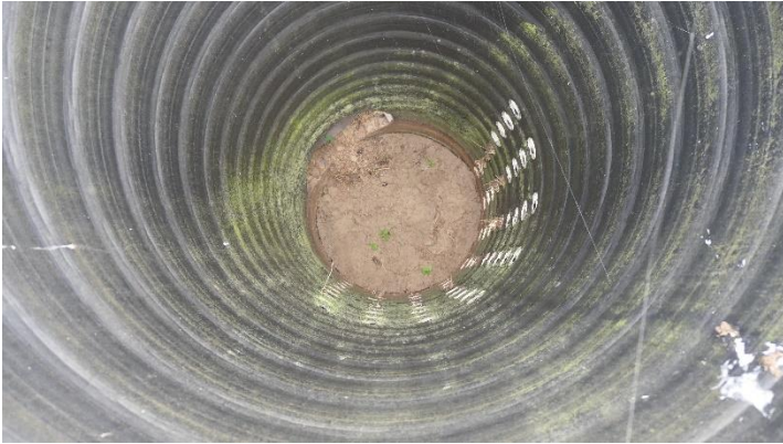
Photo 71. Inside of make-shift catch basin structure
