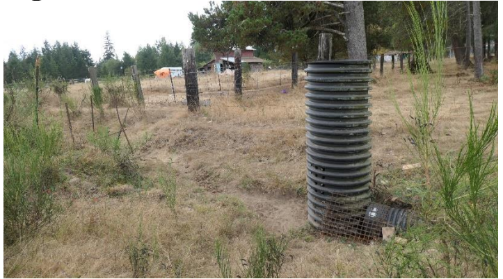
Photo 70. Ditch flows from west then to north at this structure
