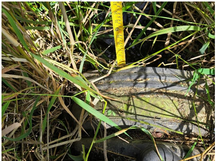
Photo 28. Corrugated Metal Pipe on Ditch Sa onsite
