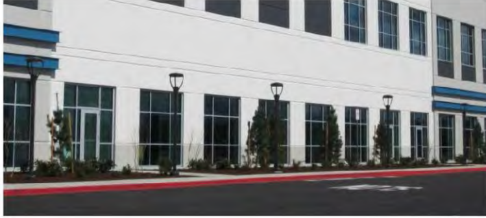
Figure 3.E.3.1-3. Lighting and landscaping help to articulate this industrial building.
