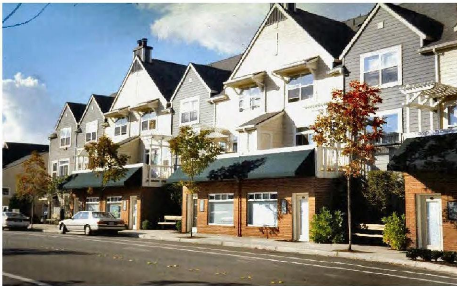
Figure 2.E.2.1-3. This mixed-use building incorporates decks, upper level setbacks, trellises, and landscaping to meet human scale guidelines.
