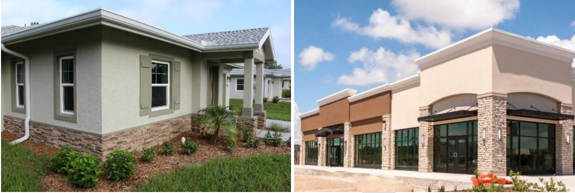
Figure 5.D.5-7. Acceptable examples of stucco finishes with roof overhangs and in conjunction with other materials.
