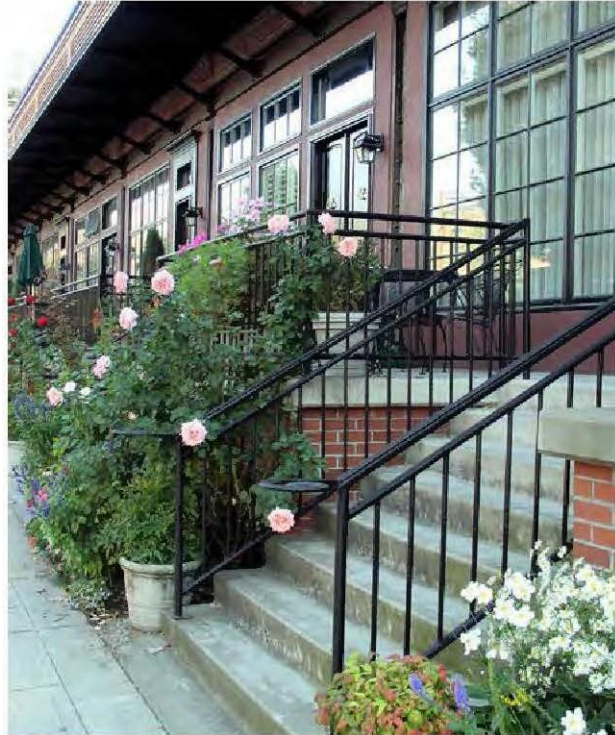
Figure 2.C.1.3-7. Raising the ground floor of residential units a few feet above grade adds privacy because pedestrians walking on the adjacent sidewalk cannot look directly into the living spaces. A small porch or stoop provides an intimate transition between public and private realms.
