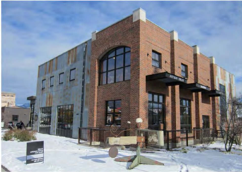
Figure 3.E.1.1-3. A successful application of approach 3: Contemporary forms and treatments. This example relates to its surroundings by using materials and colors compatible with adjacent buildings and breaking down the building's massing by providing human scale elements and articulating features..
