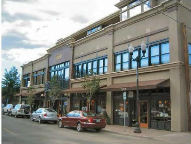
Figure 2.E.3.1-2. Example of a well-articulated building. Note how the awnings, window divisions, pilasters, columns, and cornice line all serve to divide up the façade into smaller segments without disrupting the unity of the overall design.
