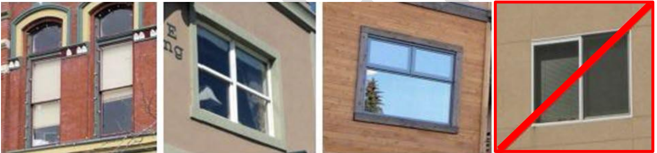
Figure 5.D.5-2. Visible window trim painted or finished in a complementary color. Note that the windows in the brick building on the left are recessed from the façade while the windows in the middle images include trim. The image on the right includes no trim or recess/projection and would not be permitted.
