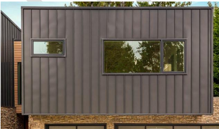
Figure 5.D.5-3. Residence with color and edge trim that cover exposed edges of sheet metal panels.
