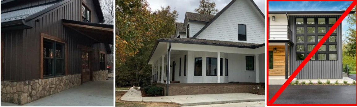
Figure 5.D.5-4. Structures with a base of stone (left) or masonry (center) extending up to at least two feet above grade. Example on the right includes metal siding all the way to the ground, which is prohibited.
