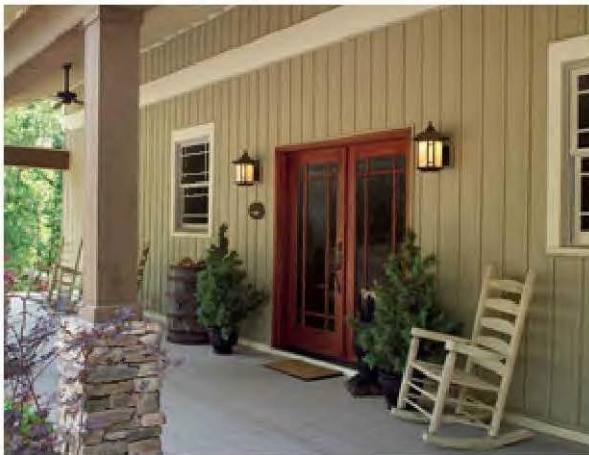
Figure 2.E.7.1-2. Fiber cement panels and similar materials are allowed when providing human scale details like this vertical siding.
