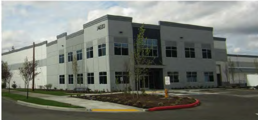
Figure 3.B.2.1-1. This building would meet the guidelines if it oriented its main entrance to the street.
