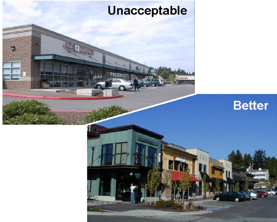
Figure 2.E.4.2-3. The continuous canopy on top is monotonous and deemphasizes individual storefronts. The bottom example provides a variety of weather protection features and represents a more desirable example.
