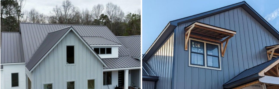
Figure 5.D.5-1. Acceptable matte finish metal siding examples in a neutral/earth tone (left example) and in a dulled blue- gray tone (right example).
