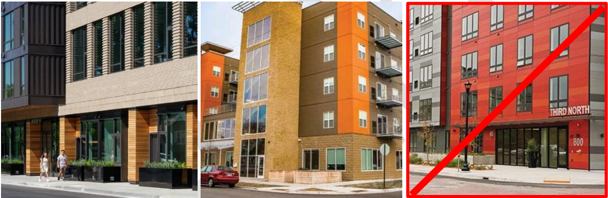
Figure 5.D.5-8. Acceptable examples illustrating the use of fiber cement panels with a different pedestrian-scale material on the ground floor façade (left and middle examples). The example on the right uses fiber cement panels on the ground floor façade, which is not acceptable.
