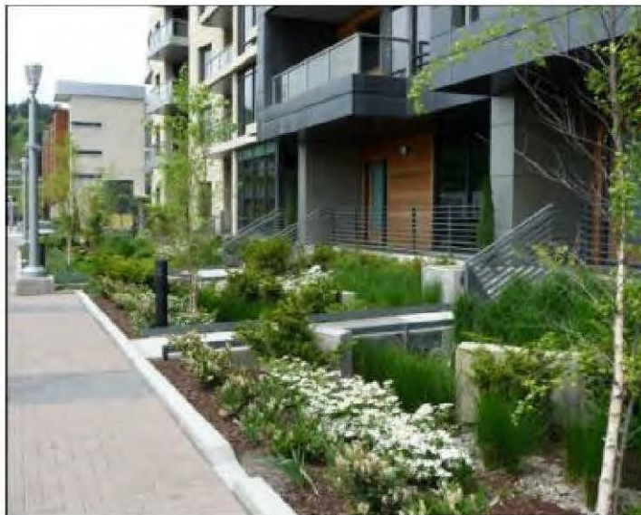
Figure 2.8.7.1-1 A preferred method of handling stormwater is through retention systems, such as rain gardens, incorporated as site amenities. Other low-impact development techniques are encouraged, and in many cases, required.
