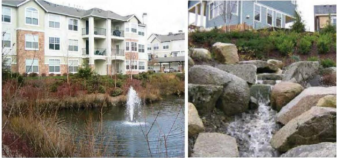
Figure 2.8.7.1-2. Example flow control system incorporated into the site design as an amenity, High Point West, Seattle
