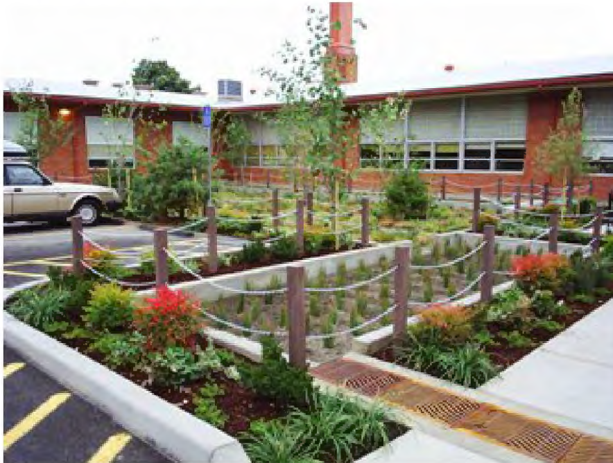
Figure 4.D.2.1-1. A Portland Middle School's parking area landscaping also serves stormwater purposes.
