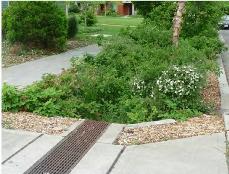
Figure 5.C.6-1. A preferred method of handling stormwater is through retention systems, such as rain gardens, incorporated as site amenities. Other low-impact development techniques are encouraged, and in many cases, required.
