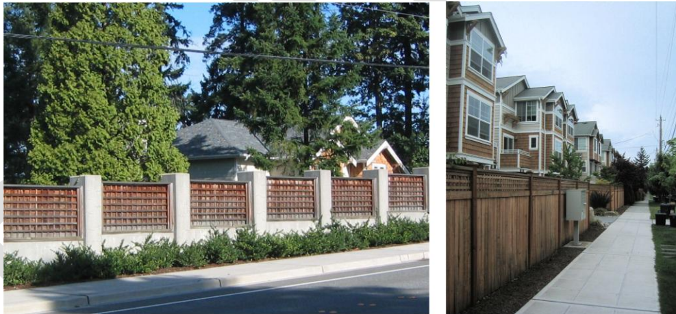
Figure 2.B.9.1-2. Fences that prevent visibility from public ROW and open spaces can decrease security.
