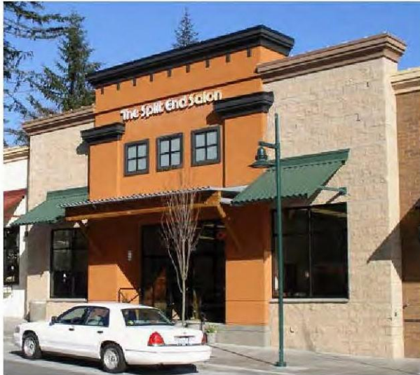
Figure 2.E.7.1-1. This storefront effectively combines stucco-like material and concrete block with wood trim and metal detailing.
