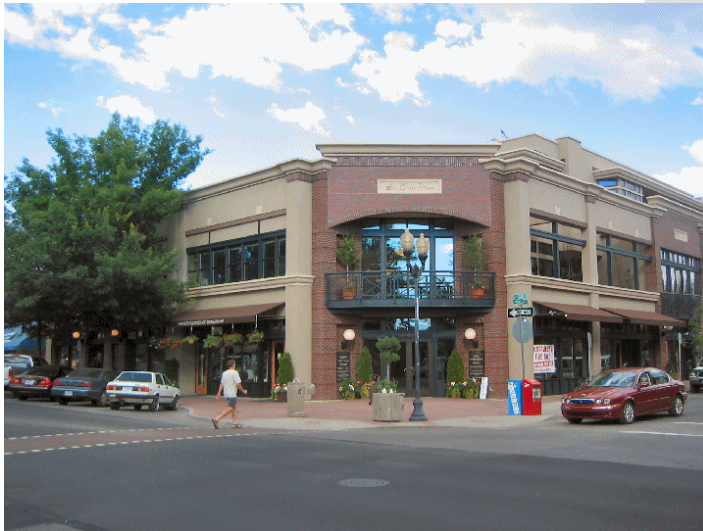
Figure 2.E.5.1-1. To emphasize its street corner location, this building uses a cropped corner, change in building materials, decorative façade elements, and a modulated roofline.
