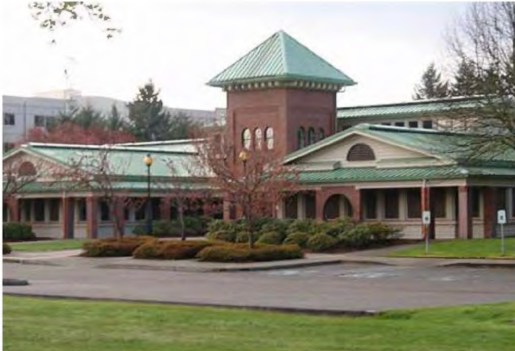
Figure 4.E.1.1-2. Tumwater City Hall exemplifies approach 2: traditional forms and materials (image: KOMO News).
