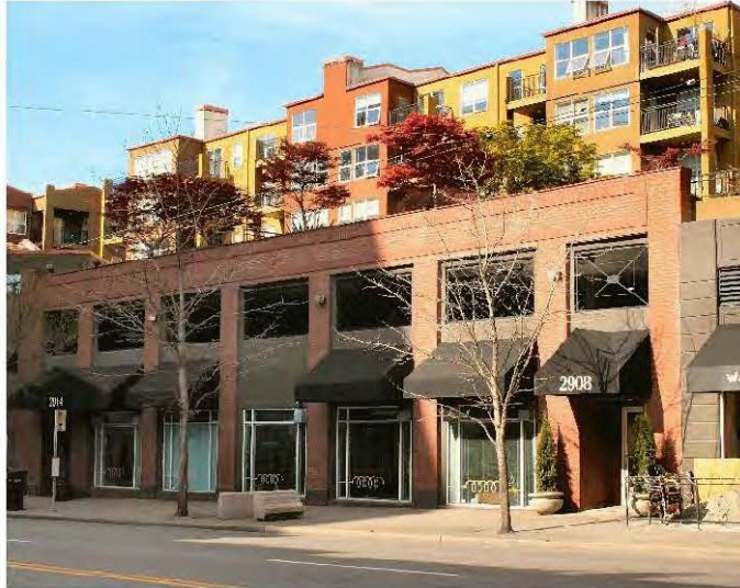
Figure 2.E.10.1-2. This building uses openings on its second level parking area to resemble windows.
