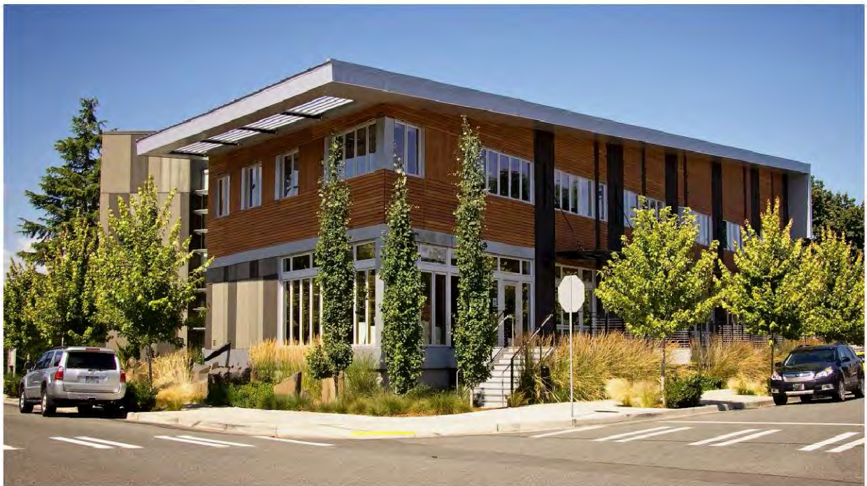
Figure 4.C.1.1-3. Snoqualmie City Hall uses landscaping that also treats stormwater between the street and building and street trees in grates to provide a pleasant pedestrian path to the entrance.
