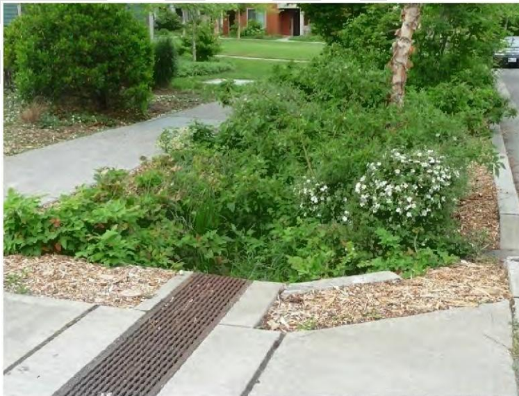
Figure 5.C.4-1. A preferred method of handling stormwater is through retention systems, such as rain gardens, incorporated as site amenities. Other low-impact development
