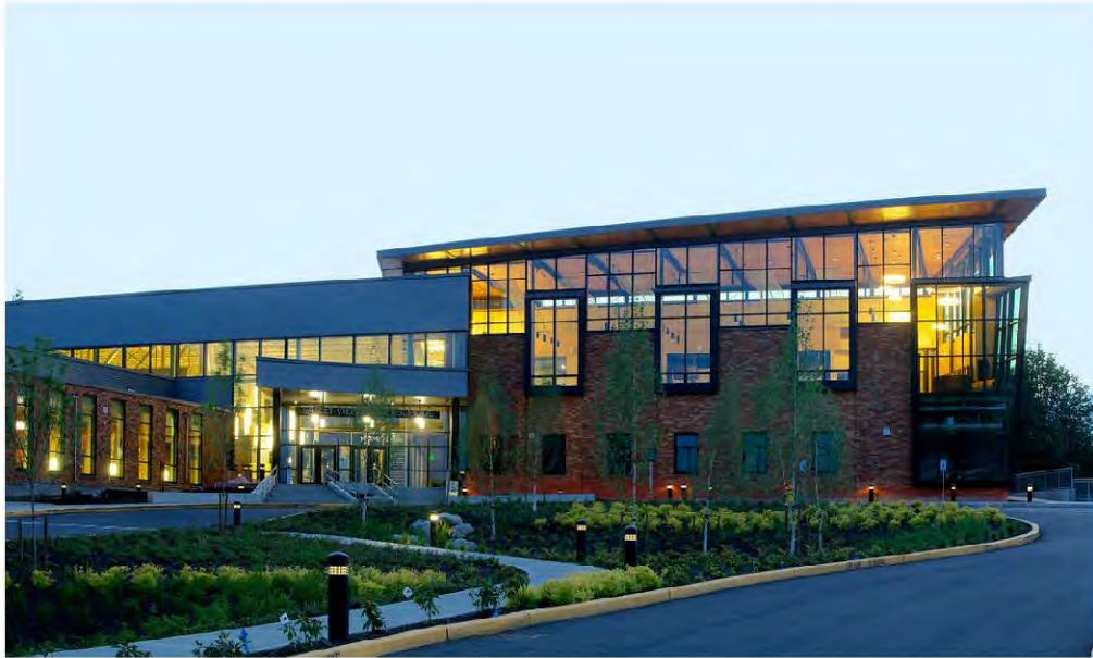
Figure 4.B.5.2-1. A preferred method of handling stormwater is through retention systems, such as rain gardens, incorporated as site amenities. Other low-impact development techniques are encouraged, and in many cases, required (image: AIA).
