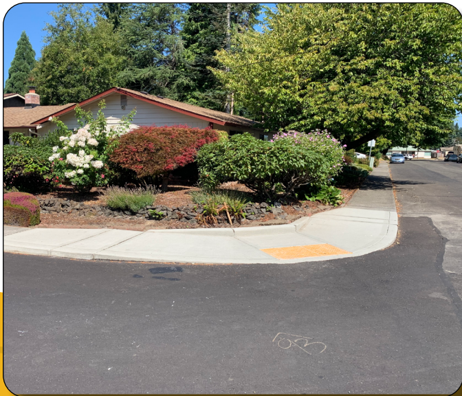
New ADA-Compliant Pedestrian Curb Ramp (2021)
