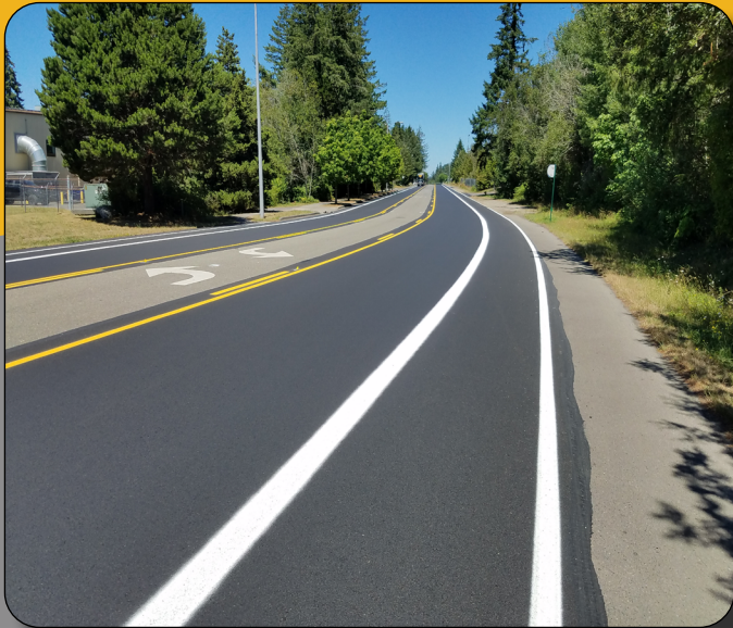
RW Johnson Blvd, Completed Mill and Inlay (2018)
