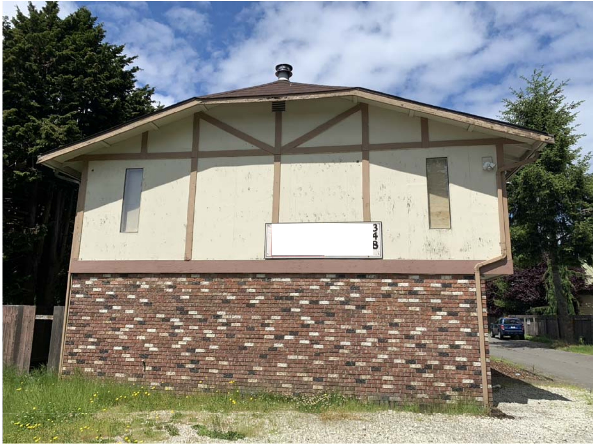
348 LEE ST SW - FACING NORTH
