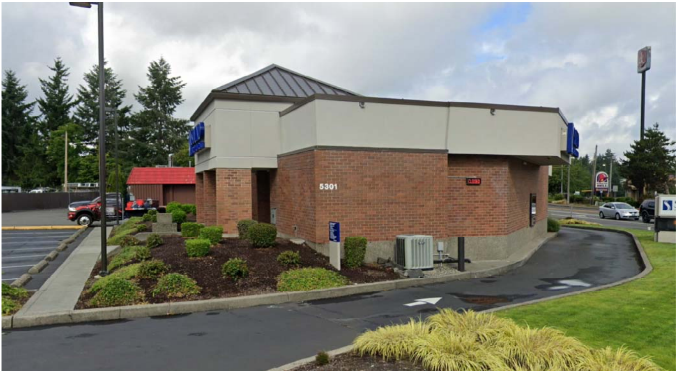
5301 CAPITOL BLVD - FACING WEST
