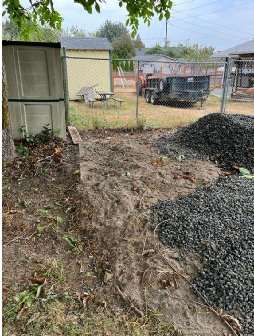
Photo of Impacts within Critical Root Zone
