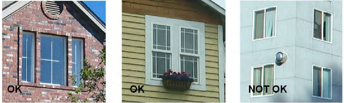
Figure 5.D.5-1 Acceptable (left and center examples) and unacceptable (right example) window treatments.
