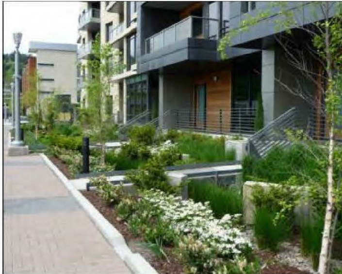
Figure 2.B.7.1-1 A preferred method of handling stormwater is through retention systems, such as rain gardens, incorporated as site amenities. Other low-impact development techniques are encouraged, and in many cases, required.
