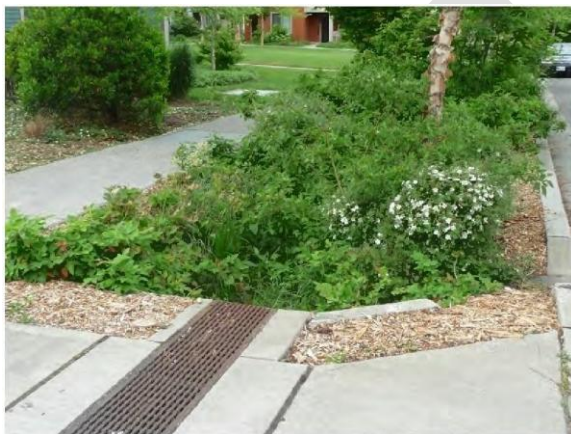
Figure 5.C.6-1. A preferred method of handling stormwater is through retention systems, such as rain gardens, incorporated as site amenities. Other low impact development techniques are encouraged, and in many cases, required.
