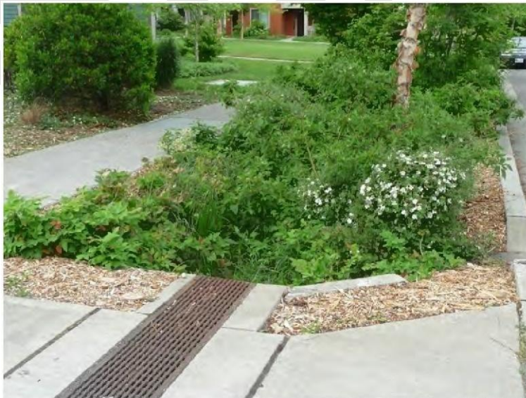
Figure 5.C.4-1. A preferred method of handling stormwater is through retention systems, such as rain gardens, incorporated as site amenities. Other low-impact development
