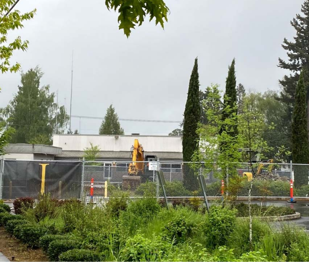
Construction on City Services Building
