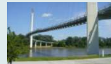
65 th Avenue Bridge
