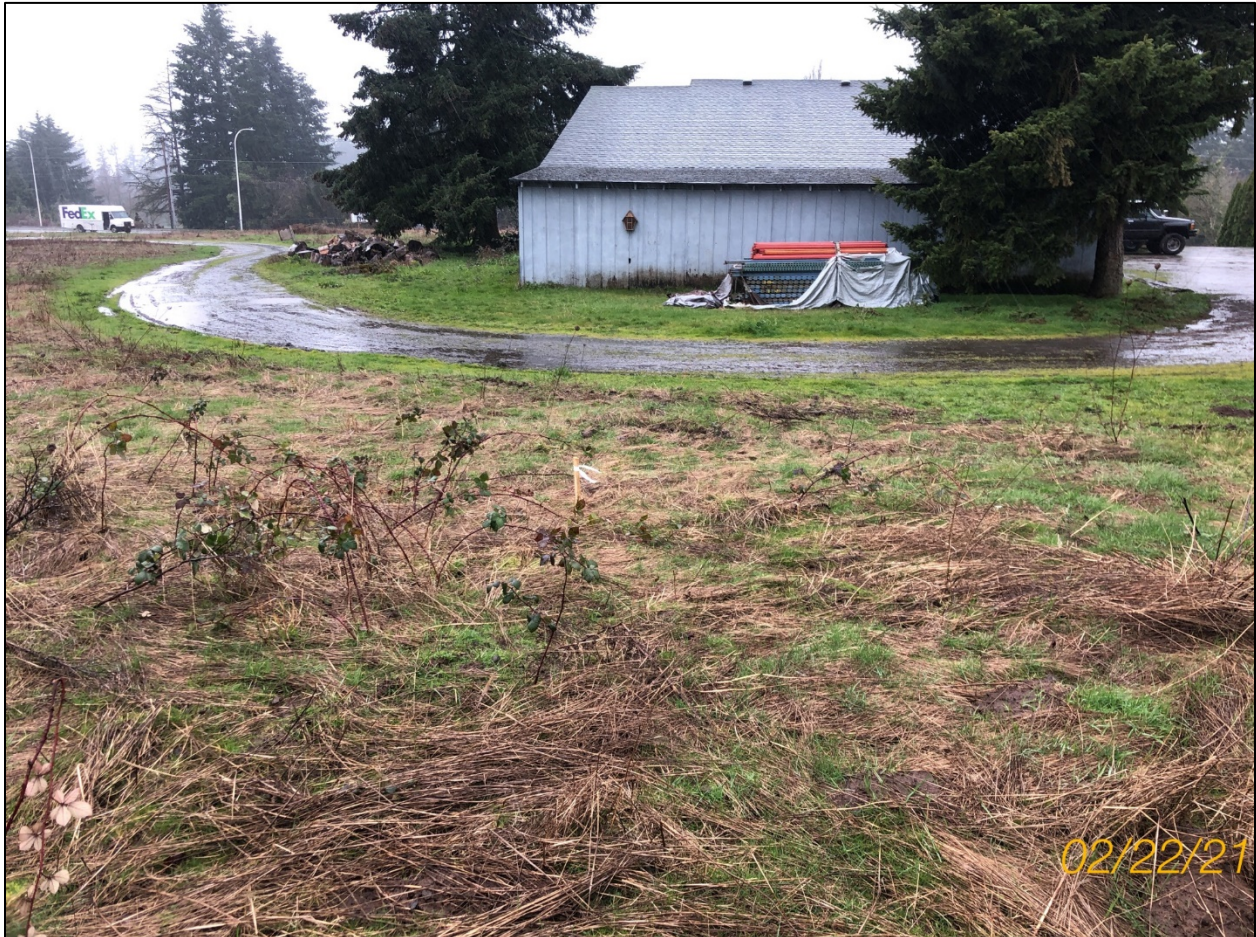
Photo 1: Looking west from the east-central portion of the site at an existing barn structure to be demolished.
