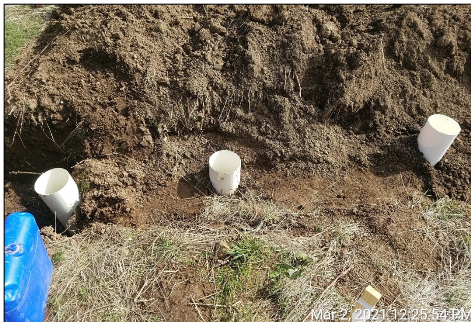
Photo 7: Backfilling around the 3 standpipes in the test pit trench at one of the infiltration test locations prior to conducting the infiltration testing.
