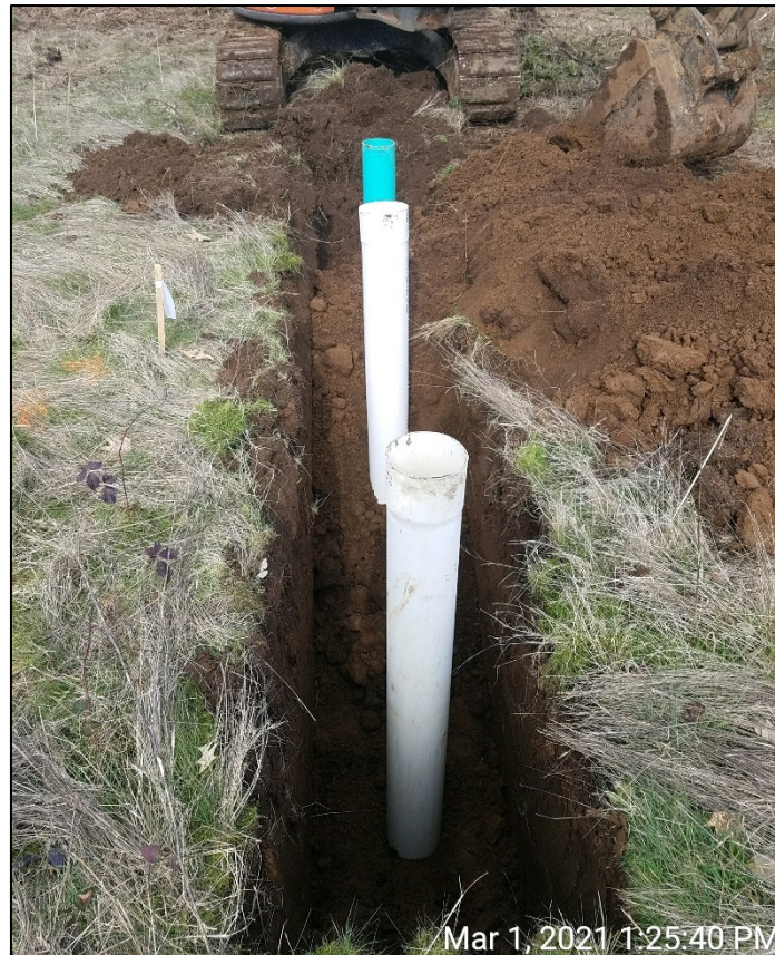
Photo 6: Setting the 3 standpipes in the test pit trench at one of the infiltration test locations.
