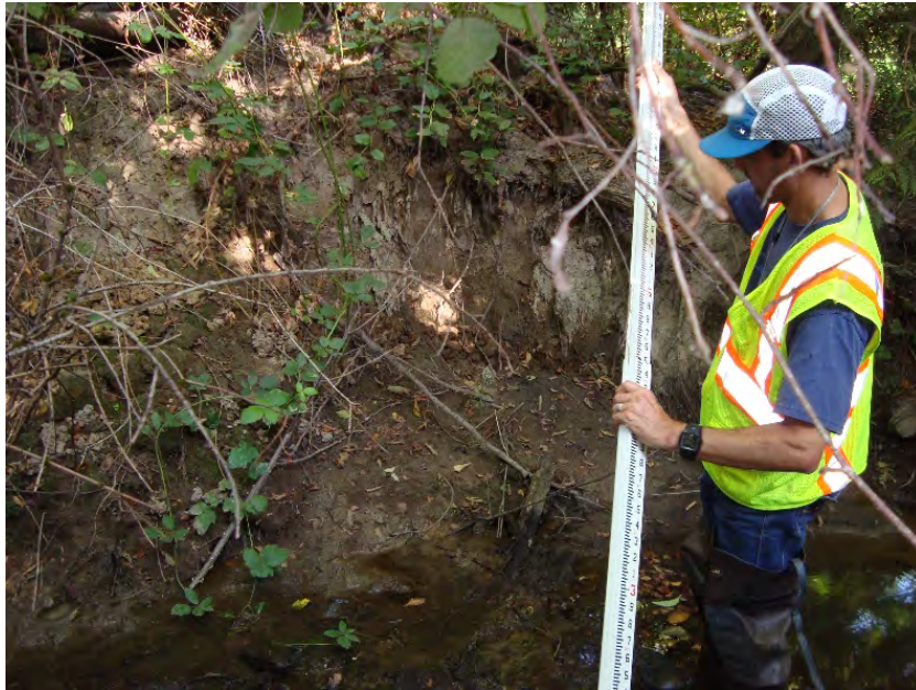
Site location: 500' upstream of confluence with S. tributary Photo number: H3-25 Description: Left bank failure, incised channel, unstable
