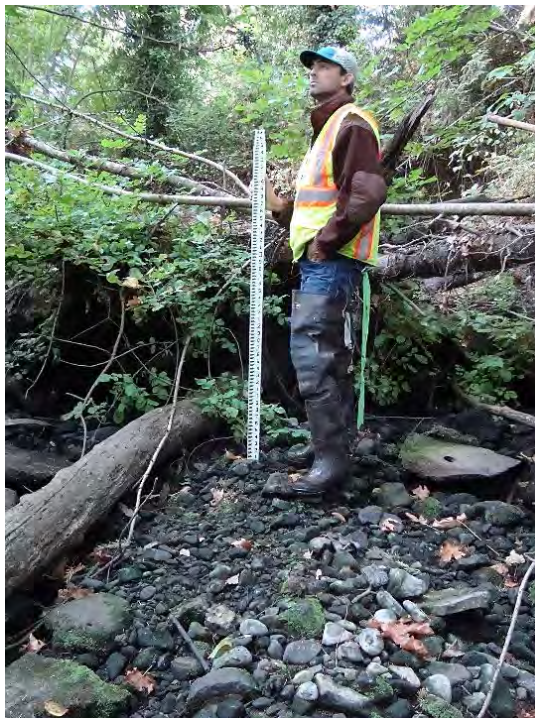
Site location: 300' upstream of Tualatin River Photo number: H1-6 Description: Looking upstream, gravel deposit in center of channel below channel-spanning debris jam
