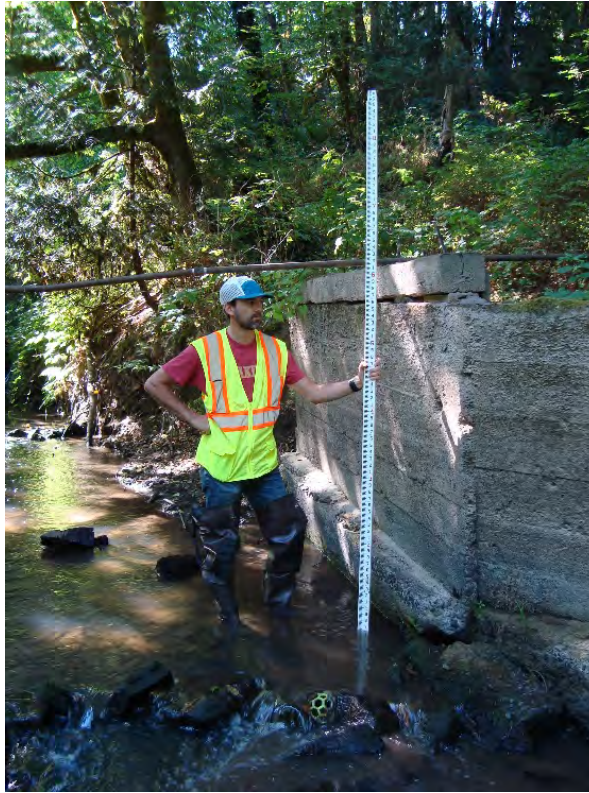
Site location: ~200' upstream from Tualatin Photo number: S1-3 Description: Former bridge abutment, looking upstream at left bank
