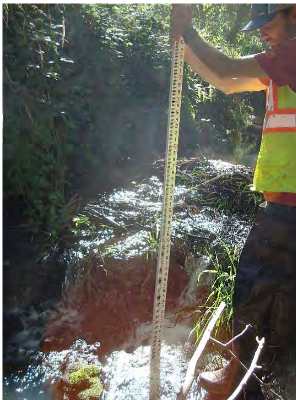
Site location: SW Prosperity Park Rd culverts Photo number: S1-22 Description: Looking upstream at twin 36" culverts
