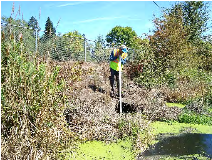
Site location: Upstream side of SW Nyberg Lane Photo number: N1-3 Description: Looking downstream at culverts, same location as Photo N1-2
