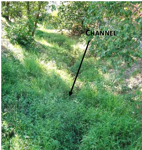
Photo 7. Nyberg Creek Reach #3 upstream of SW Martinazzi Avenue.
