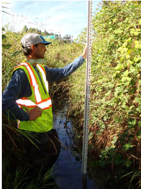
Site location: South of SW 59th Photo number: S2-10 Description: Location of 12" steel pipe in channel disconnected from vertical segment. Some gravel in channel at this location.
