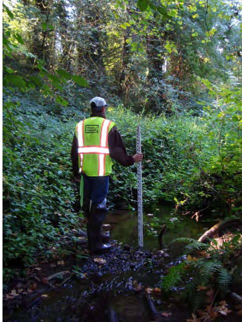
Site location: 30' upstream of SW 105 th Ave. Photo number: H3-3 Description: Right bank hillslope failures, wetland plants growing on slope (wet)
