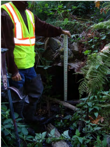
Site location: Culvert at SW 105 th Ave. (upstream side) Photo number: H3-2 Description: Looking downstream at SW 105 th Ave. culvert crossing from east side of SW 105 th Ave.
