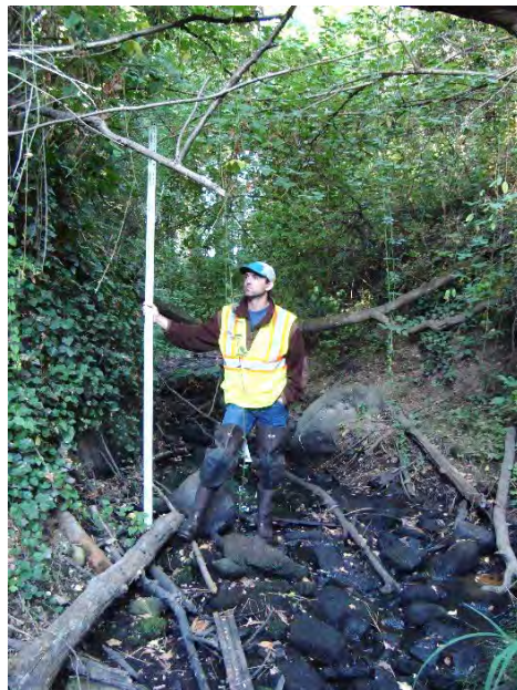
Site location: 30' upstream of Tualatin River Photo number: H1-2 Description: 1' - 2' rocks in channel, high water mark on bridge abutment corresponds to about 6' above channel bed in this location, steep gradient to mouth
