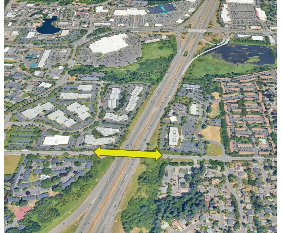
Sagert St Bridge Pedestrian Facility (see also Nyberg Creek Trail)
