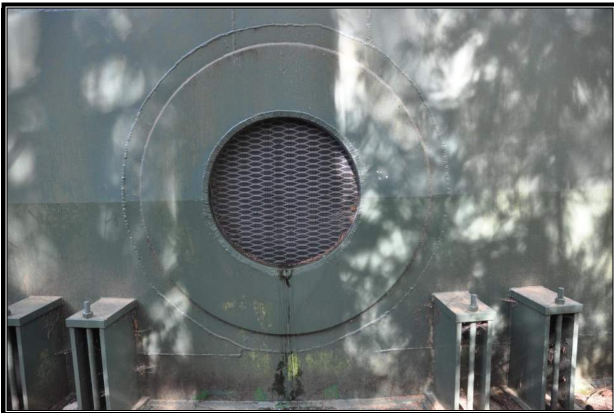
2.2 MG A1 Reservoir – Overflow Discharge
