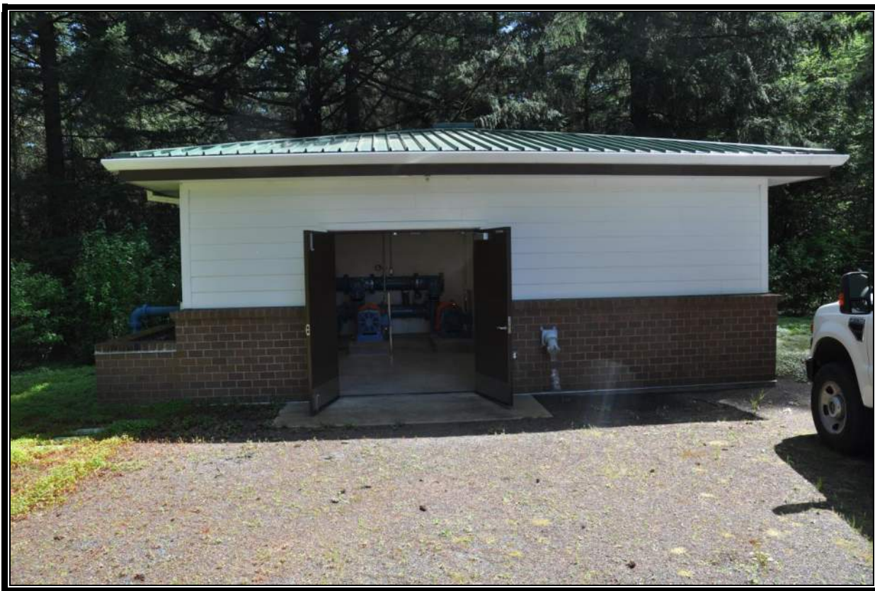
C Level Norwood Pump Station
