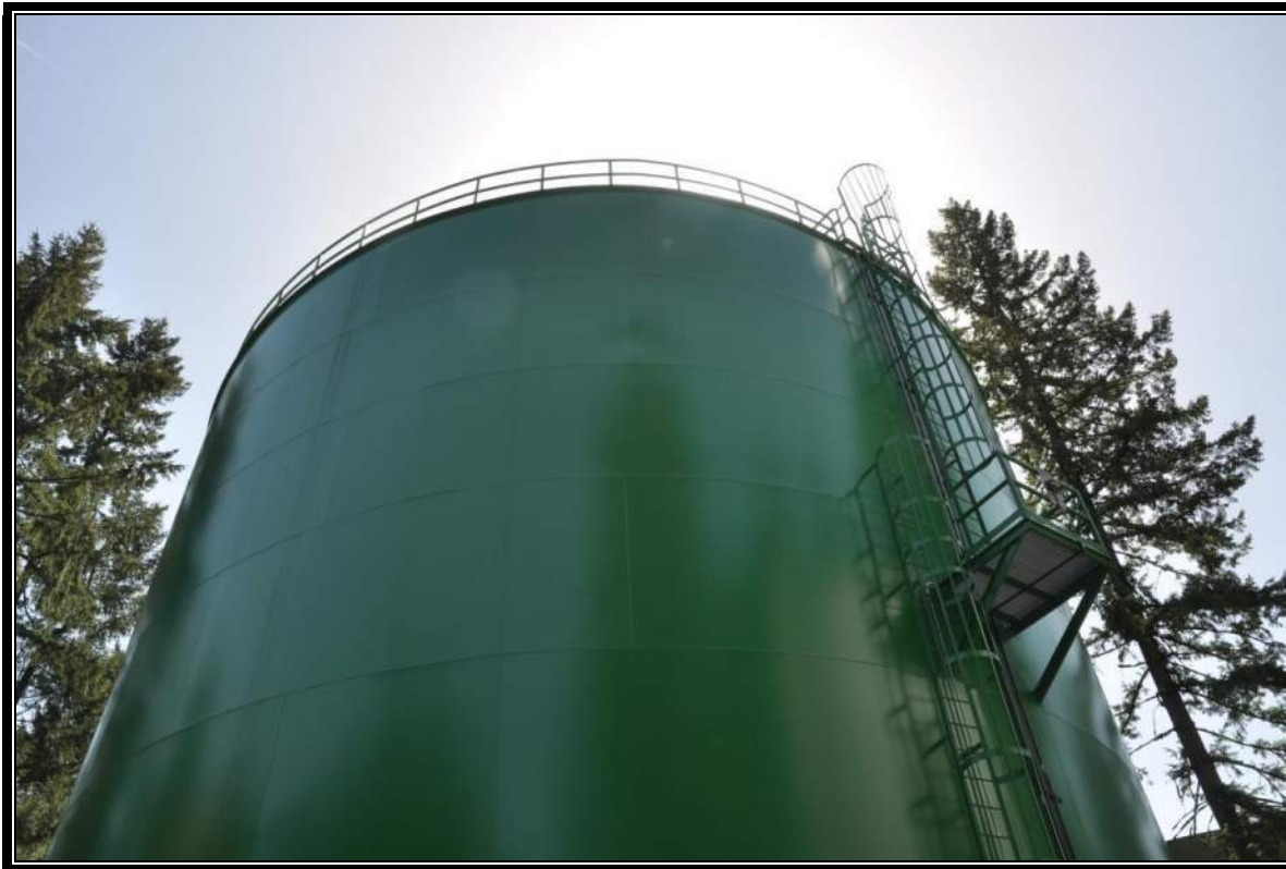
1.0 MG C2 Reservoir – Wall Shell Plates
