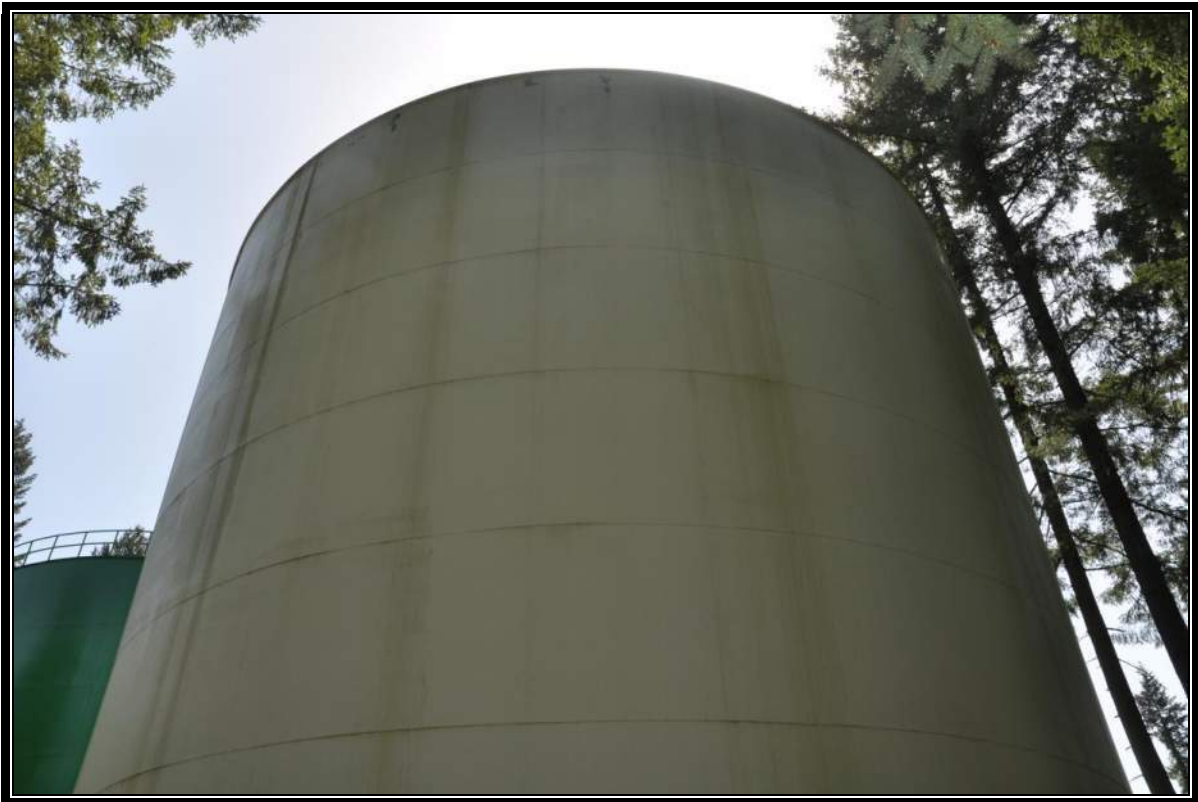
0.8 MG C1 Reservoir – Wall Shell Plates
