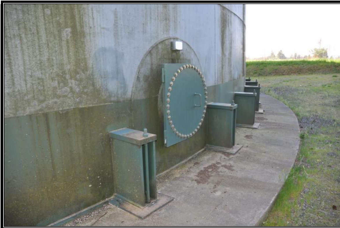
2.2 MG B2 Reservoir – Anchorage Retrofit
