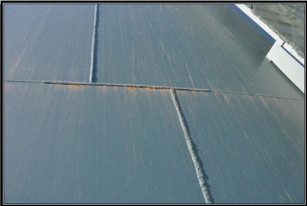
5.0 MG A2 Reservoir – Wall Shell Welds
