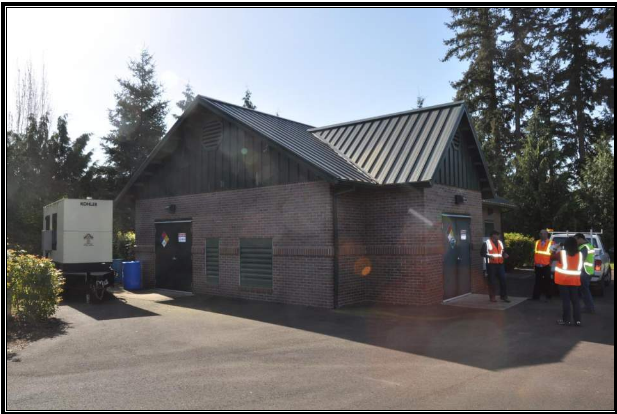
ASR Pump Station
