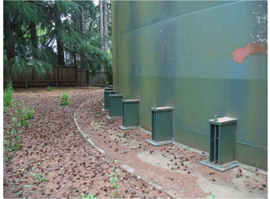
Photo 4: A-1 Reservoir, foundation and structure elements (May 30, 2018).
