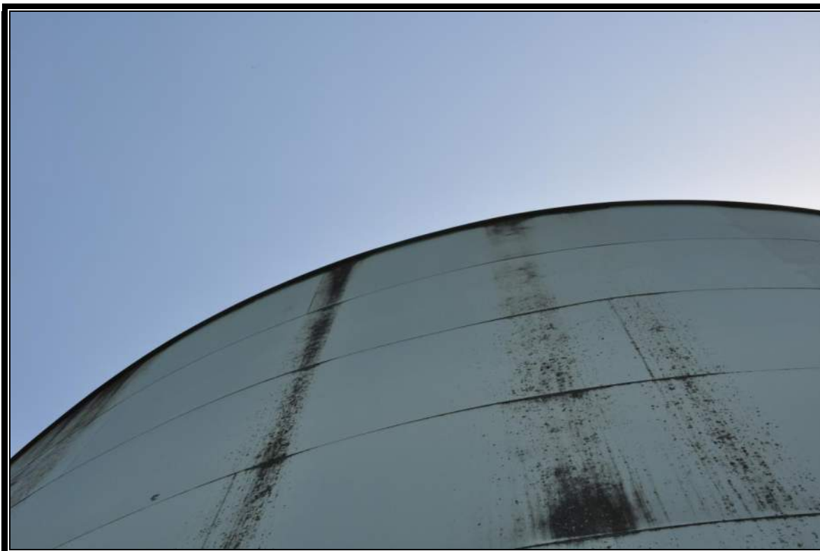
2.2 MG B2 Reservoir – Wall Shell Plates
