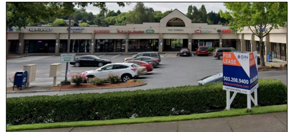
Nyberg Retail Center: 7052 SW Nyberg Street
