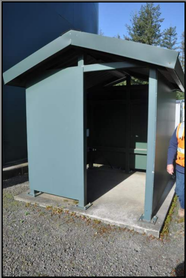
5.0 MG A2 Reservoir - Shelter
