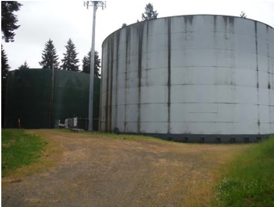
Photo 5: Norwood reservoirs and pump station, looking south (May 30, 2018).
