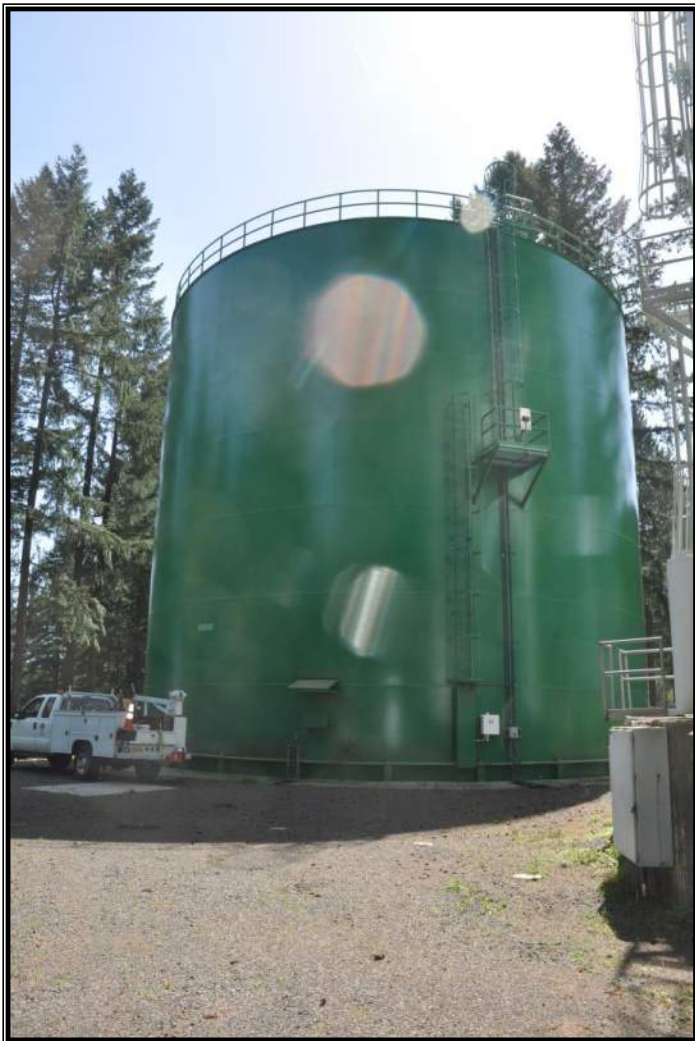
1.0 MG C2 Reservoir
