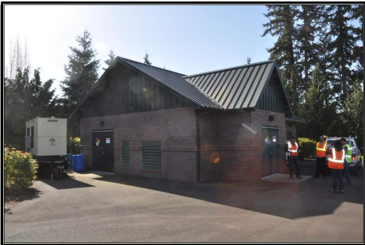
ASR Pump Station
