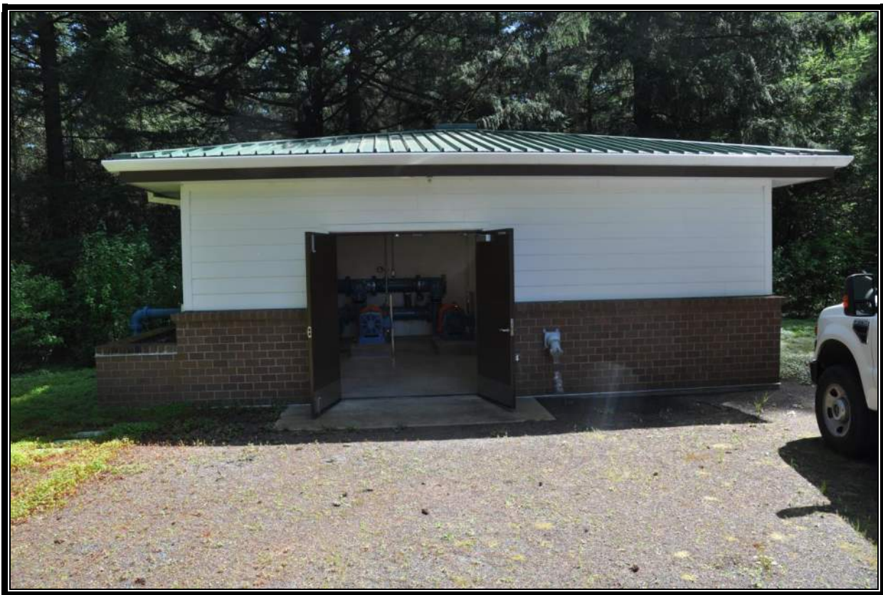
C Level Norwood Pump Station
