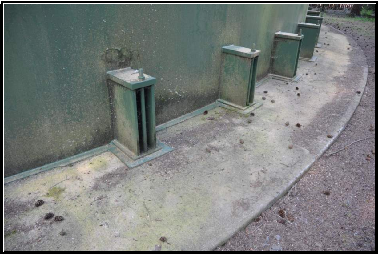
2.2 MG A1 Reservoir – Foundation and Anchorage Retrofit
