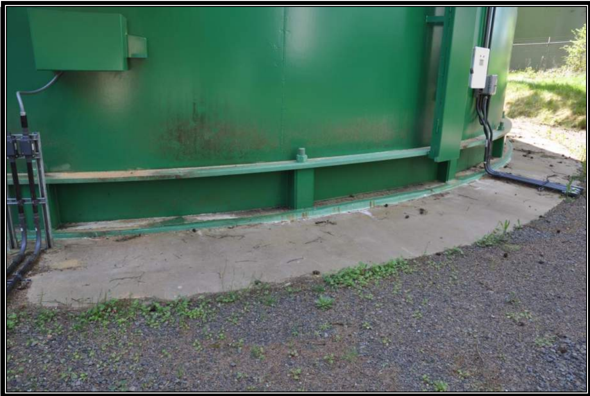
1.0 MG C2 Reservoir – Anchors and Foundation
