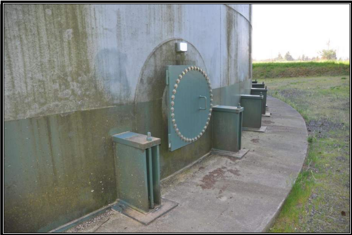
2.2 MG B2 Reservoir – Anchorage Retrofit
