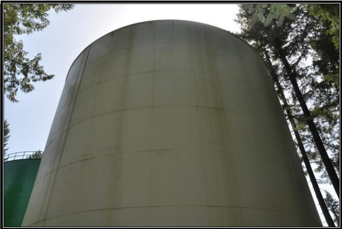
0.8 MG C1 Reservoir – Wall Shell Plates
