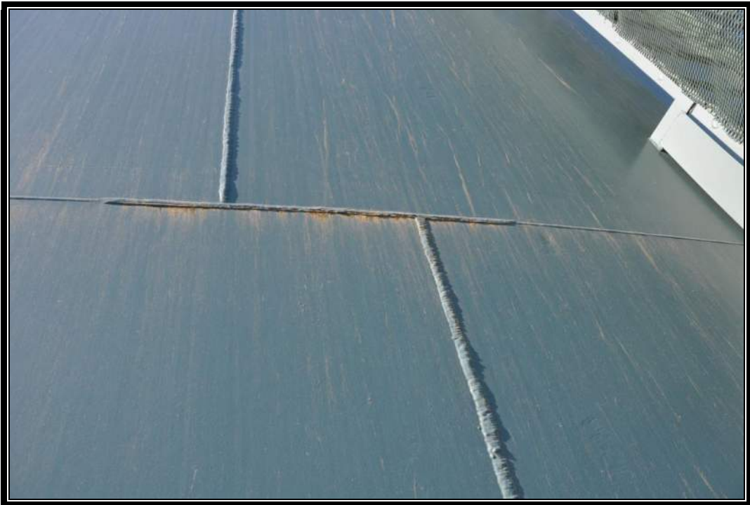
5.0 MG A2 Reservoir – Wall Shell Welds
