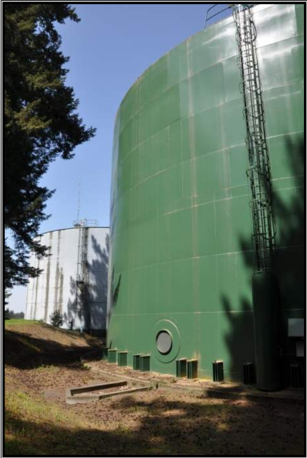
2.2 MG B1 Reservoir – Overflow Discharge and Catch Basin
