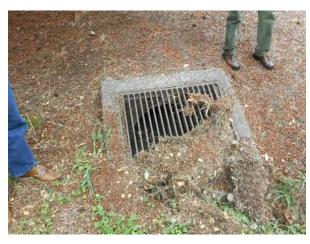
Image 2. Tree debris clogging the ditch inlet at the downstream end of the open channel
