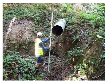
Image 1. Perched outfall from Blake Street with severe bank failure
