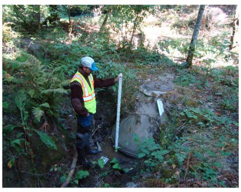
Image 1. Location 'M' exposed sanitary manhole and incised tributary
