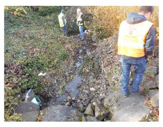
Image 2. Accumulated ballast and debris upstream of culverts across Boones Ferry Road
