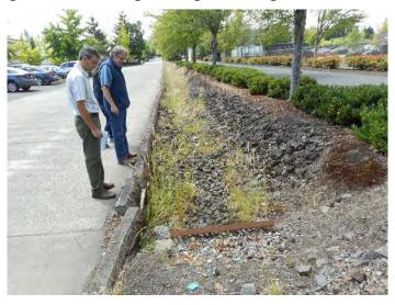
Image 2. Grated inlet and rock lined channel at downstream end of drainage ditch
