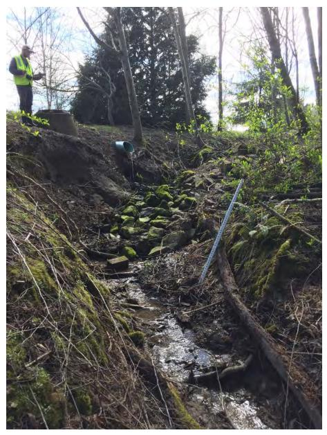
Image 2. Location 'N' outfall and channel erosion (photo provided by OTAK)
