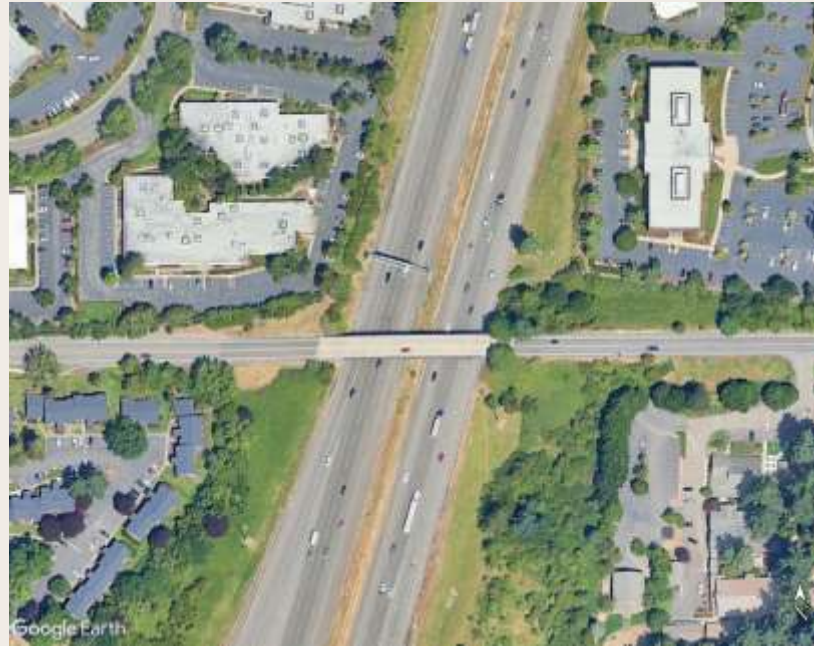
Sagert Street Bridge Lights
