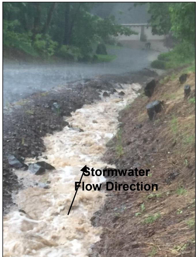
**Photo A2c.** The junction for the ditch and driveway pipe are overwhelmed and flood waters drain into the front yard toward the house (5-18-15).
