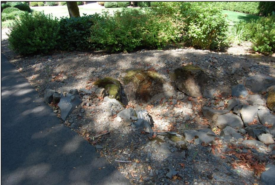
**Photo A3d.** This photo of the westernmost base of the ditch was taken on August 19, 2016 and looks generally west toward the Lucini house. Shown the basin where stormwater collects and is routed into the entrance of the 12-inch corrugated plastic pipe (CPP), which is visible in the center of the photo. This pipe entrance allows flows to go south into the driveway culvert. Although a reversed view, this photo corresponds to the flood location in Photo A2c of the previous Appendix A2.
