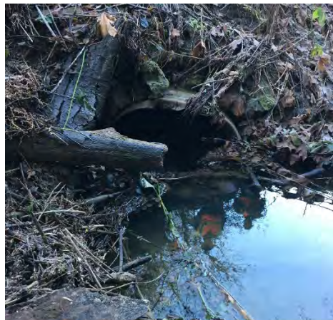
Image 2. Upstream end of culvert
