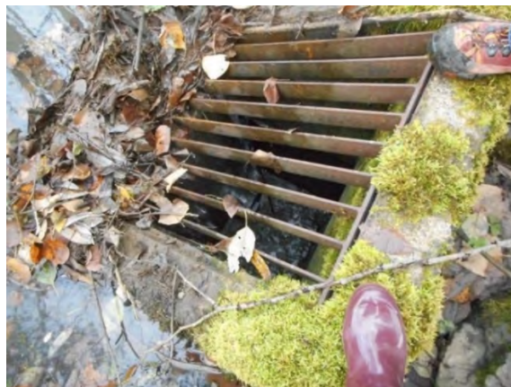
Image 2. Existing pond outfall control structure
