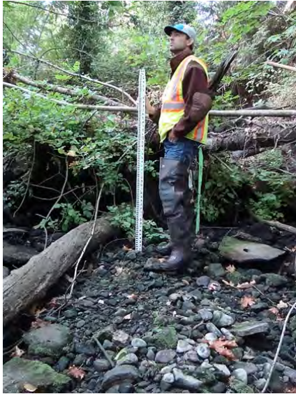
Channel-spanning debris jam in Hedges Creek Reach #1 approx. 300' upstream of Tualatin River (photo location shown below with camera icon)
