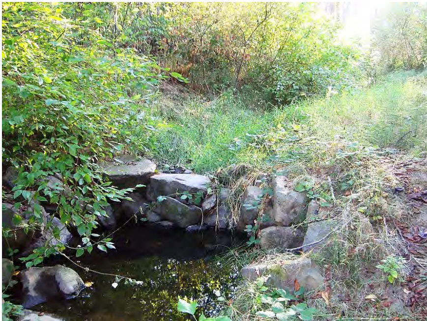
Site location: ~350' upstream of SW Blake St. Photo number: S3-8 Description: Constructed rock pool
