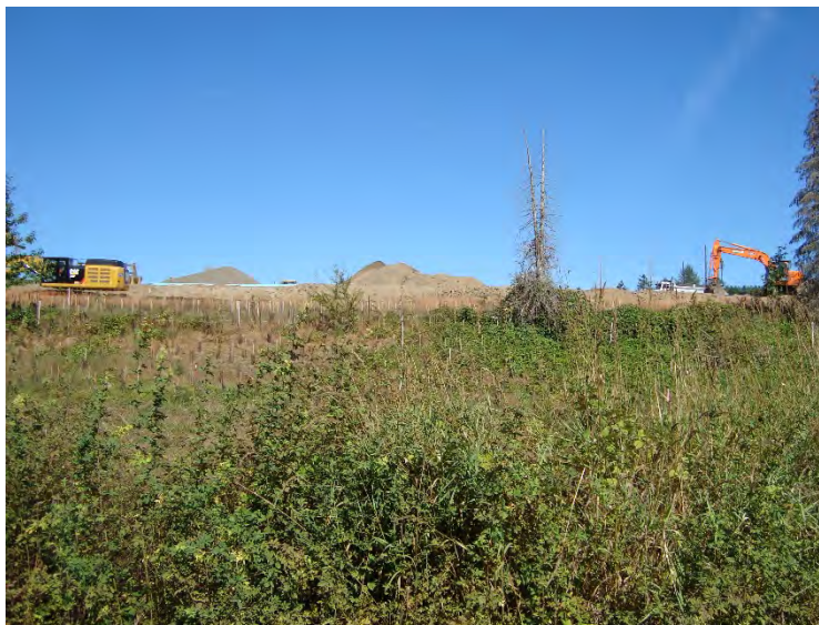
Site location: 1000' east of SW 65 th Ave. Photo number: S2-16 Description: Looking north at construction site across channel
