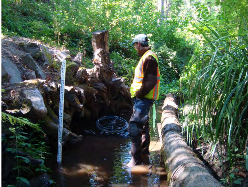
Site location: 950' upstream of SW 105 th Ave. Photo number: H3-15 Description: Restoration area, looking downstream. Left bank root wads, right bank anchored log
