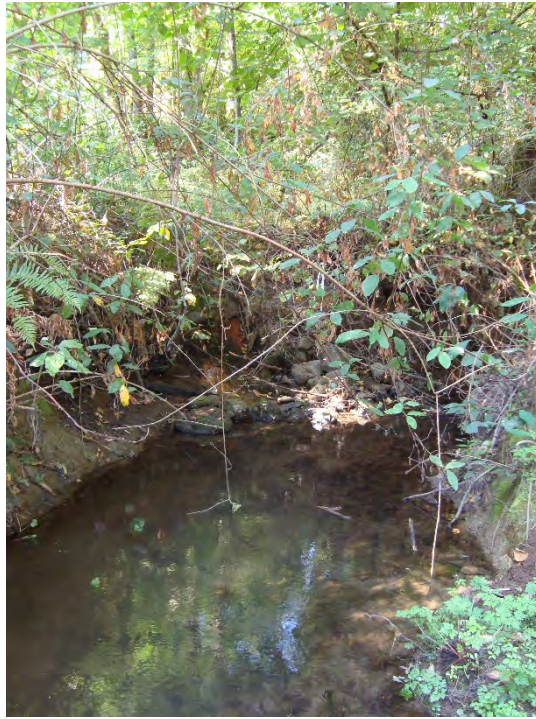
Site location: 800' upstream of SW 105 th Ave. Photo number: H3-13 Description: Looking downstream at outside bend, eroding left bank
