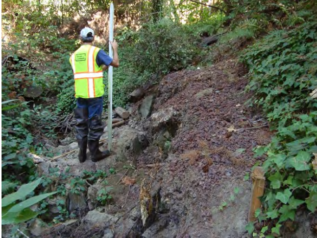
Unstable hillslope and debris in channel. Photo Location shown below with camera icon.
