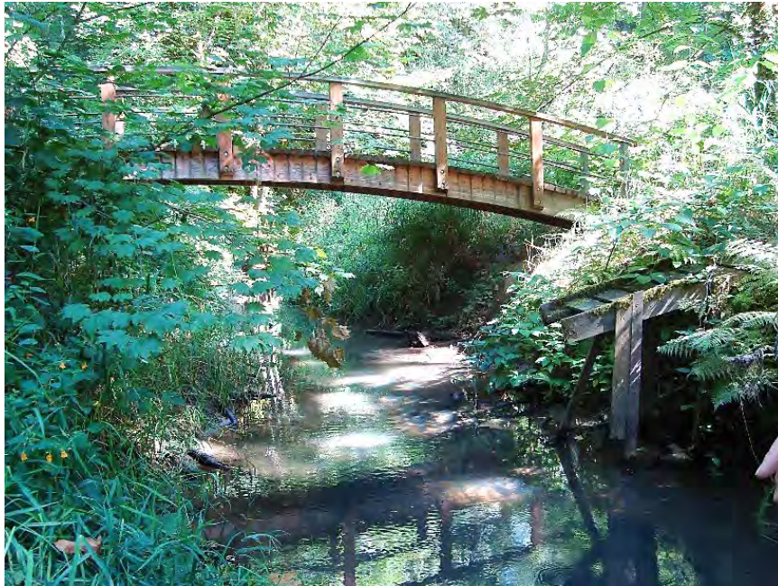
Site location: ~1,200' downstream from SW Borland Rd. Photo number: S1-15 Description: Pedestrian bridge looking upstream, silty bed
