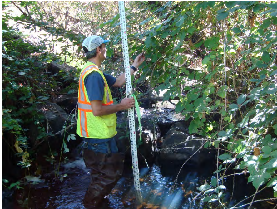
Site location: 100' downstream from SW Industrial Way Photo number: H2-13 Description: Rock drop pool formed by rip-rap energy dissipation at culvert outfall
