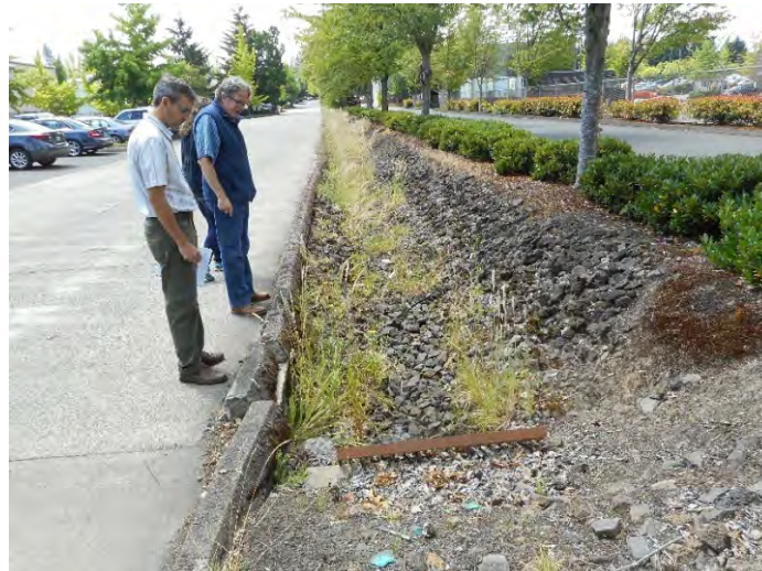
Image 2. Grated inlet and rock lined channel at downstream end of drainage ditch
