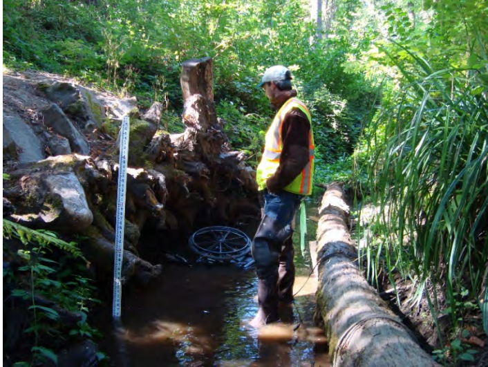
Photo 13. Restoration area showing cabled logs and root wads. Approximately 950 feet upstream of SW 105th Avenue.
