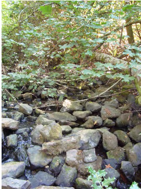
Site location: Immediately downstream from confluence with S. tributary Photo number: H3-21 Description: Looking upstream, riprap
