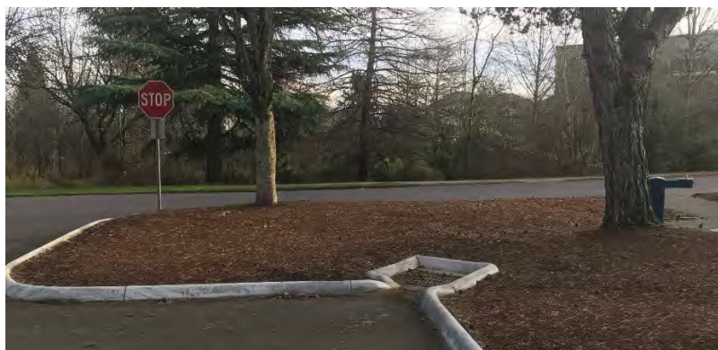
Image 2. Proposed location for Water Quality Facility #2
