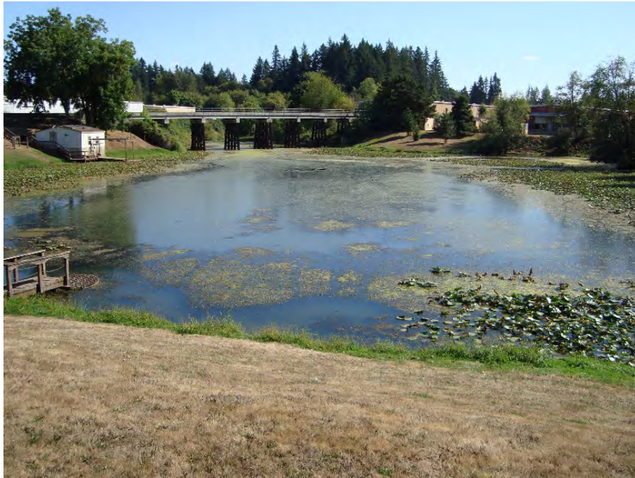
Site location: Upstream side of SW Industrial Way Photo number: H2-15 Description: Fire pond #1 in-line with Hedges Creek
