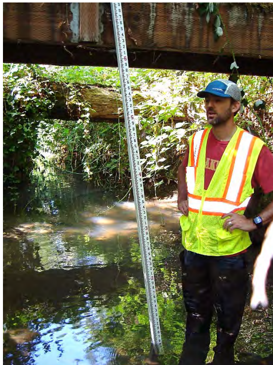
Site location: ~1,200' downstream from SW Borland Rd. Photo number: S1-16 Description: Pedestrian bridge looking downstream, large tree down across channel in distance
