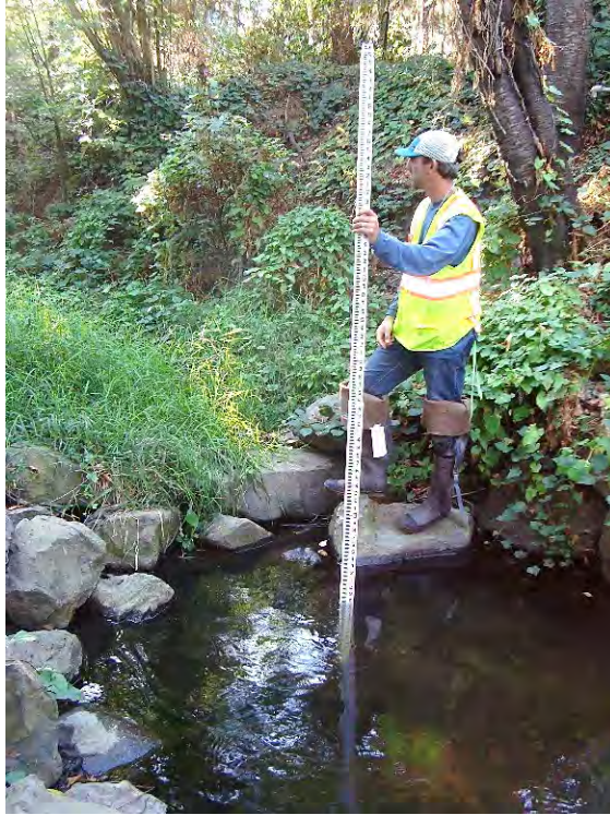
Site location: ~300' upstream of SW Blake St. Photo number: S3-7 Description: Constructed rock drop pool (restoration)
