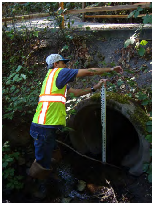
Site location: Culvert crossing under trail Photo number: H3-22 Description: Looking downstream, confluence with tributary from the south
