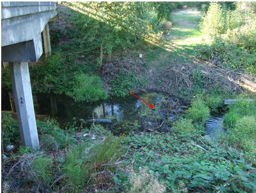
Site location: Nyberg Creek on downstream side of SW 65 th Ave (east side) Photo number: N1-12 Description: Photo taken from south side on 9/11. Red arrow shows debris removed from beaver activity.
