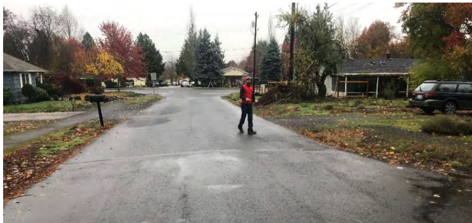
Image 1. Roadside ditches and unimproved roadway at the north end of 93 rd Avenue
