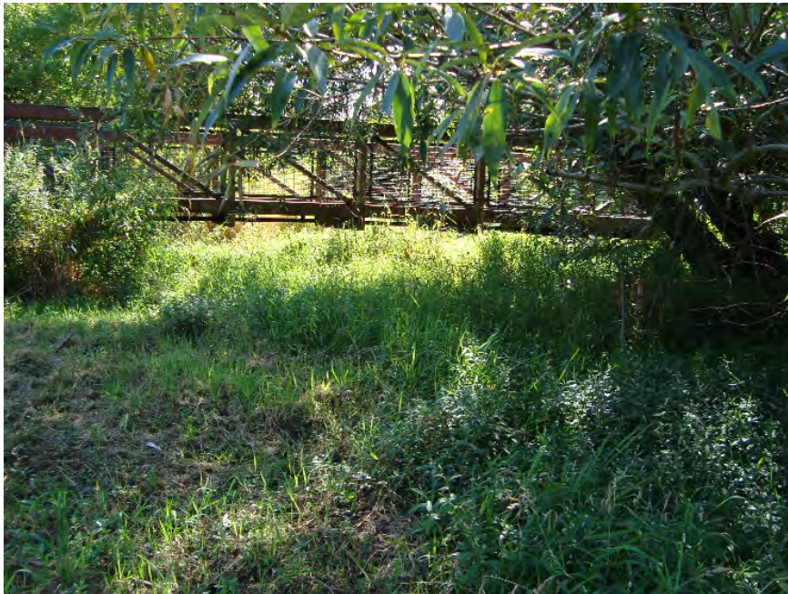
Site location: 200' downstream of SW Tualatin Road Photo number: H1-22 Description: Pedestrian bridge in wetland area downstream of SW Tualatin Road.
