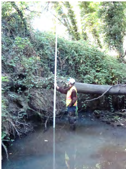
Site location: 150' upstream of Tualatin River Photo number: H1-4 Description: Looking upstream, right bank erosion, downed trees, slumping on right bank
