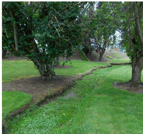
Image 1. Incision and sloughing in the open channel
