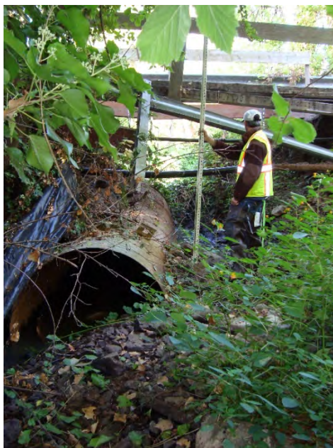
Photo 8. Culvert placed in debris from washed out bridge to convey Hedges Creek.
