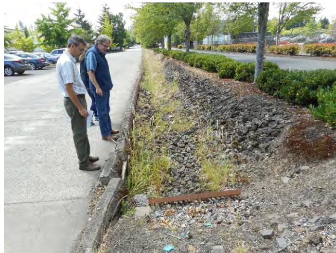
Image 2. Grated inlet and rock lined channel at downstream end of drainage ditch
