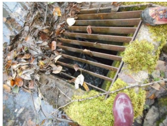
Image 2. Existing pond outfall control structure
