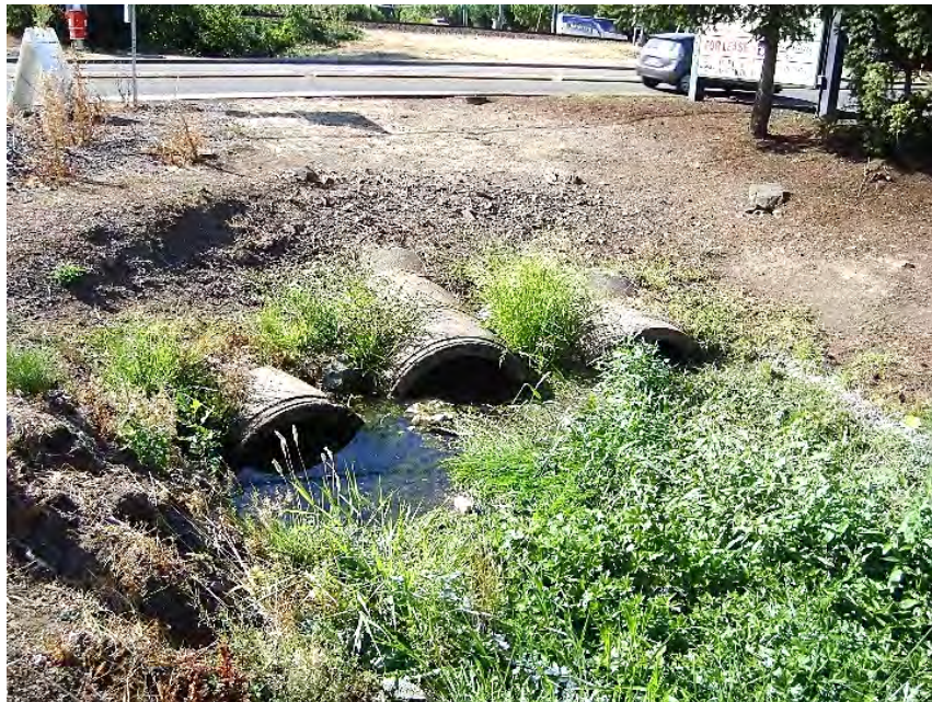
Site location: SW Boones Ferry Rd. Photo number: N3-10 Description: Culverts entering Nyberg Creek from SW Boones Ferry Rd.
