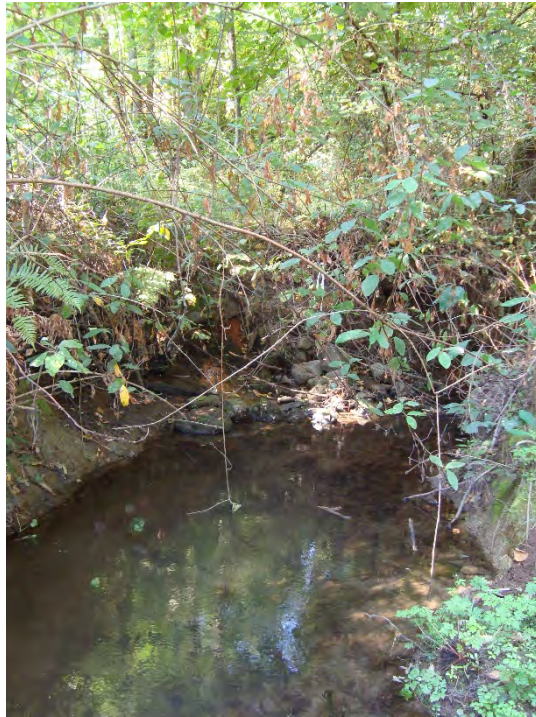
Site location: 800' upstream of SW 105 th Ave. Photo number: H3-13 Description: Looking downstream at outside bend, eroding left bank
