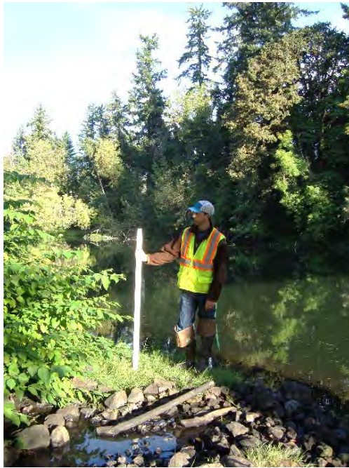
Site location: Mouth of Hedges Creek below Boones Ferry Road bridge at Tualatin River Photo number: H1-1 Description: 3" to 1.5' rocks in channel (rip-rap stabilization)
