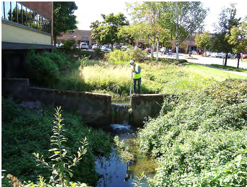
Site location: Upstream of SW Martinazzi Ave. by Shari's restaurant Photo number: N3-2 Description: Nyberg Creek, concrete dam with notch
