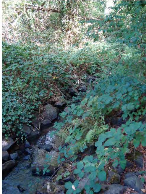
Site location: Culvert at SW Tualatin-Sherwood Road Photo number: H2-1 Description: Armored channel with rip-rap, looking downstream
