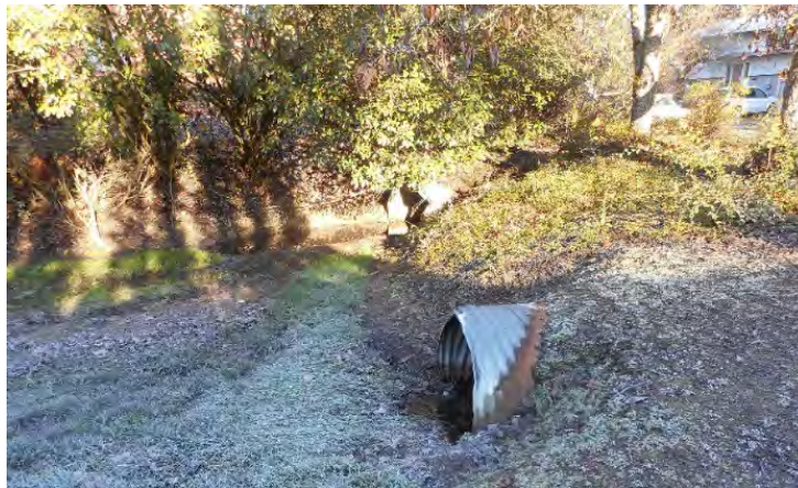
Image 1. Existing outfalls to Siuslaw Lane Greenway
