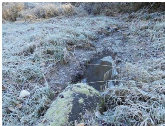
Image 2. Sediment deposition near outfall of stormwater system
