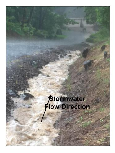
**Photo A2c.** The junction for the ditch and driveway pipe are overwhelmed and flood waters drain into the front yard toward the house (5-18-15).
